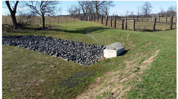
*Photos, clockwise from upper left: A vegetative filter strip planted to trap sediments and other pollutants in runoff; a water and sediment control basin installed to help control erosion and runoff, and a restored wetland that improves water quality by trapping and filtering runoff while creating a diverse habitat for wildlife.*
