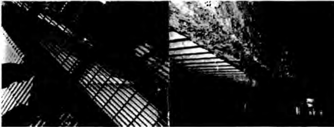
Figure 6 Membrane Tank Structural Steel Rusting
