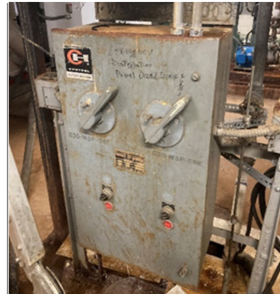
Fig P-29 Sump Pump Control Panel
