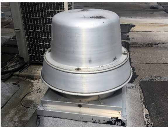
Fig H-9 - Typical Toilet Exhaust Fans
