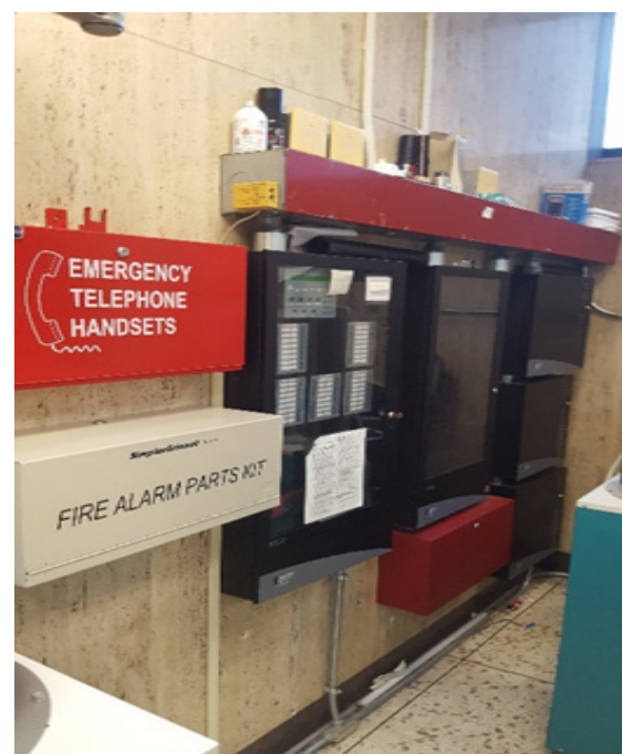
Fig E-14 - Fire Alarm System Control Panel
