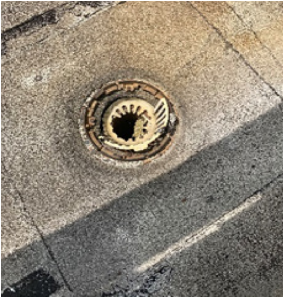
Fig P-27 - Roof Drain
