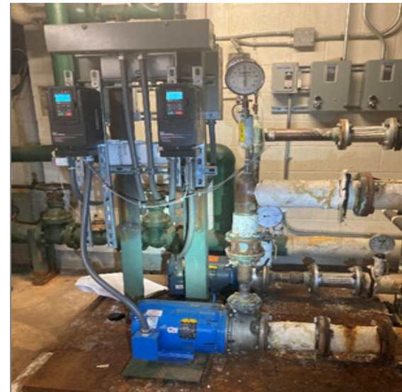
Fig P-2 - Domestic Water Dual Booster Pump System
