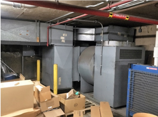
Fig H-3- Garage Exhaust Fans
