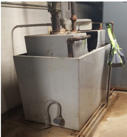
Fig E-12 - Generator Fuel Tank Cut Open and Drained
