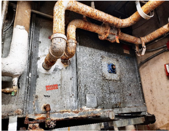
Fig H-13 - Air Handling Unit Corrosion
