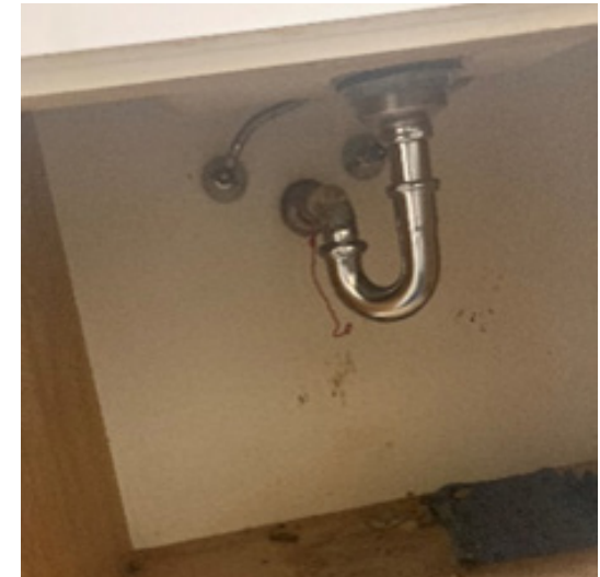
Fig P-26 - Kitchen Sink Drain Assembly
