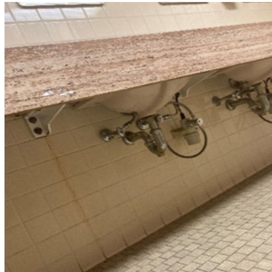
Fig P-18 - Lavatory Drain Assembly
