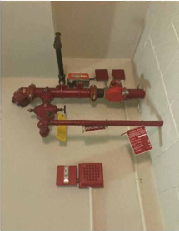
Fig P-35 - Wet Floor Control Valve
