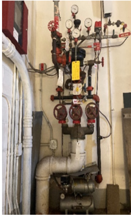
Fig P-36 - Preaction Valve and Standpipe Manifold
