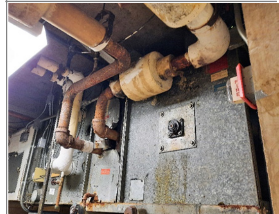
Fig. H-1 - Typical Air Handling Units
