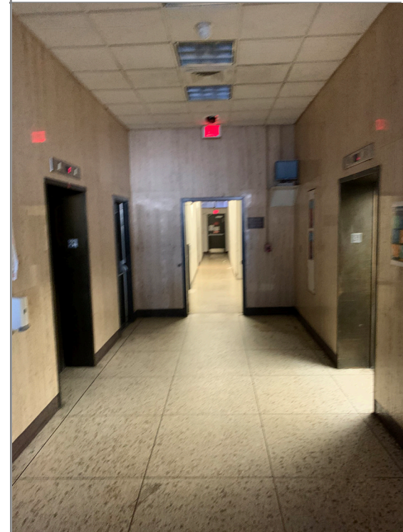
First floor elevator lobby. In general, the elevator lobby on each floor will need to be enclosed with fire rated assemblies.
