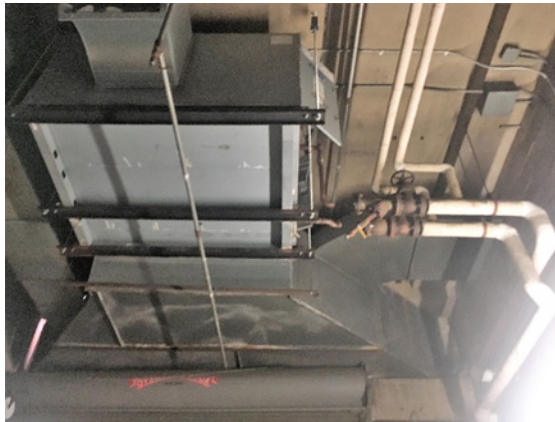
Fig H-4 - Garage Heating & Ventilating Unit
