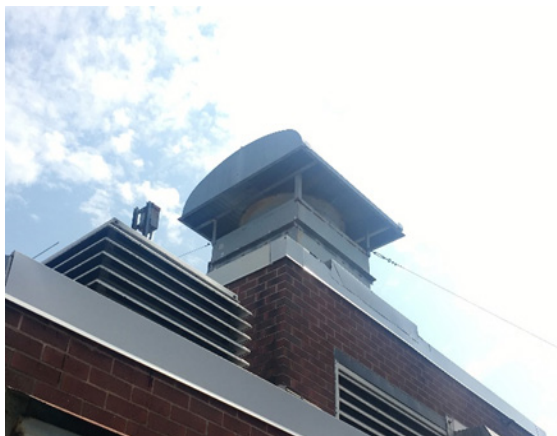
Fig H-10 - Typical Stairway Pressurization Fans
