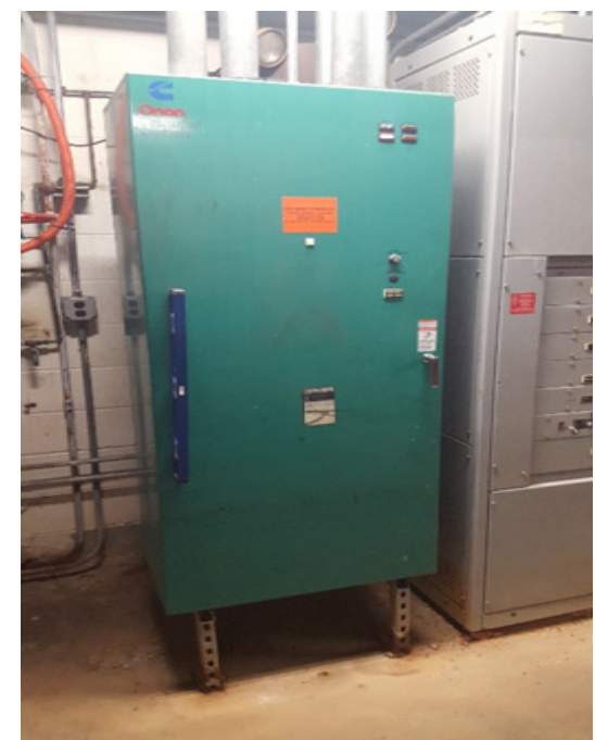
Fig E-13 - Emergency, Automatic Transfer Switch
