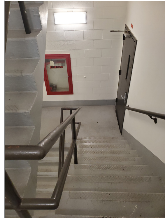
Typical egress stair with standpipe. The existing vertical enclosure meets the 2 hr fire rating requirement. Handrails and guardrails need to be upgraded to meet current codes.
