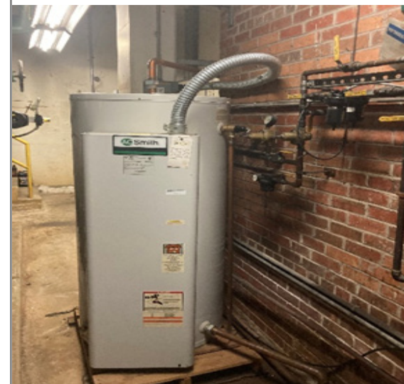
Fig P-3 Electric Water Heater
