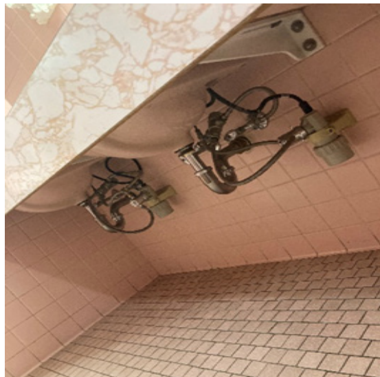
Fig P-13 - Lavatory Drain Assembly
