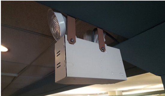
Fig E-8 - Unite Battery Light Mounted Below ADA Height
