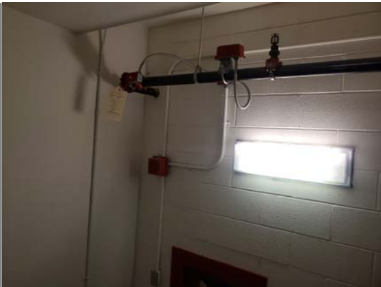
The existing fire sprinkler system and other fire protection systems will need to be reconfigured and upgraded to accommodate the building uses and to meet current code requirements.
