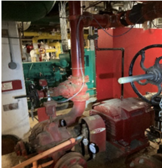
Fig P-31 - Fire Pump
