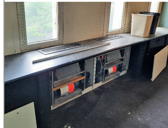
Fig. H-2 - Typical Fan Coil Units
