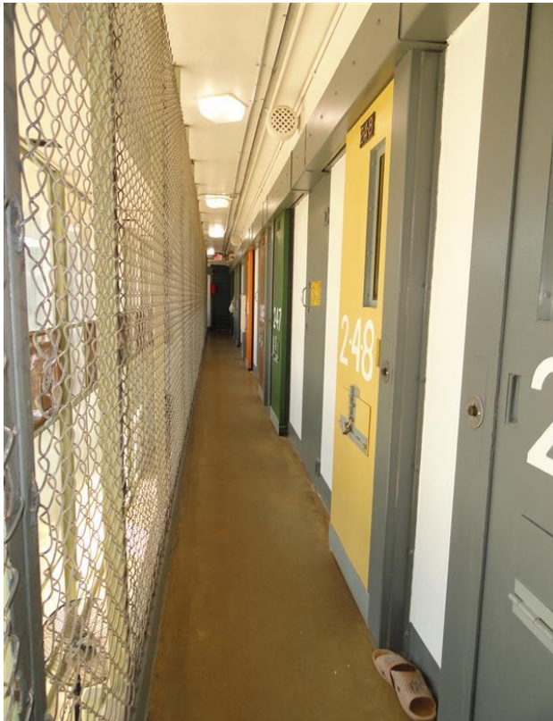
Bayside State Prison, housing unit, second floor view down the tier. Photograph by Office of the Corrections Ombudsperson, October 7, 2025.
