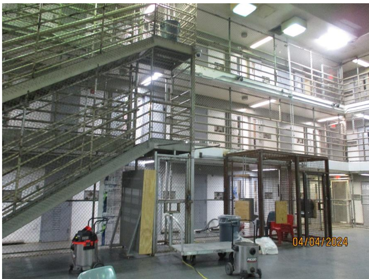
Three tiers of cells in an RHU wing at Northern State Prison and individual cages for accessing the phone and kiosk. Photograph taken by Office of the Corrections Ombudsperson, April 4, 2024.
