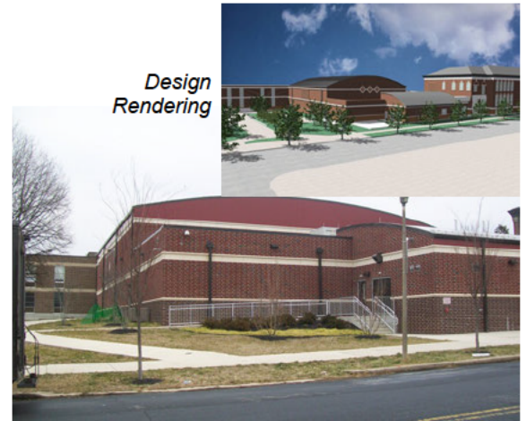
Penrose ES & Motivation HS Gymnasium & Cafeteria Addition, School District of Philadelphia
