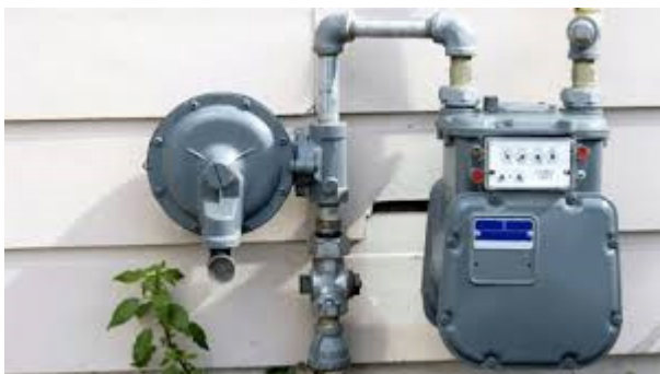
Figure D-15 A typical meter set with a relief valve. John Lewis.
