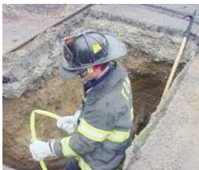
Figure D-19 Never enter a trench/excavation without proper training and NEVER attempt to kink a flowing gas line. Lee Calderio.
