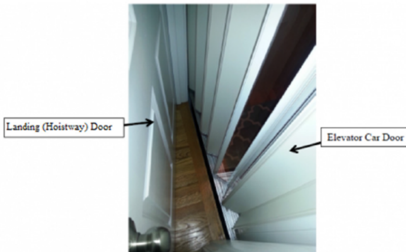
Typical Private Residence Elevator with Exterior Landing (Hoistway) Door and Interior Elevator Car (Accordion) Door
