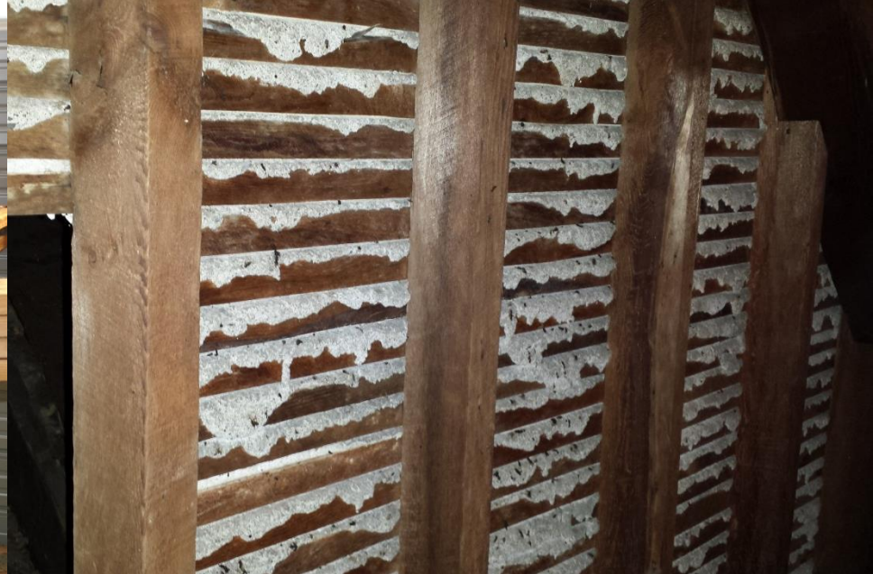
Guano visible on lath & plaster attic walls
