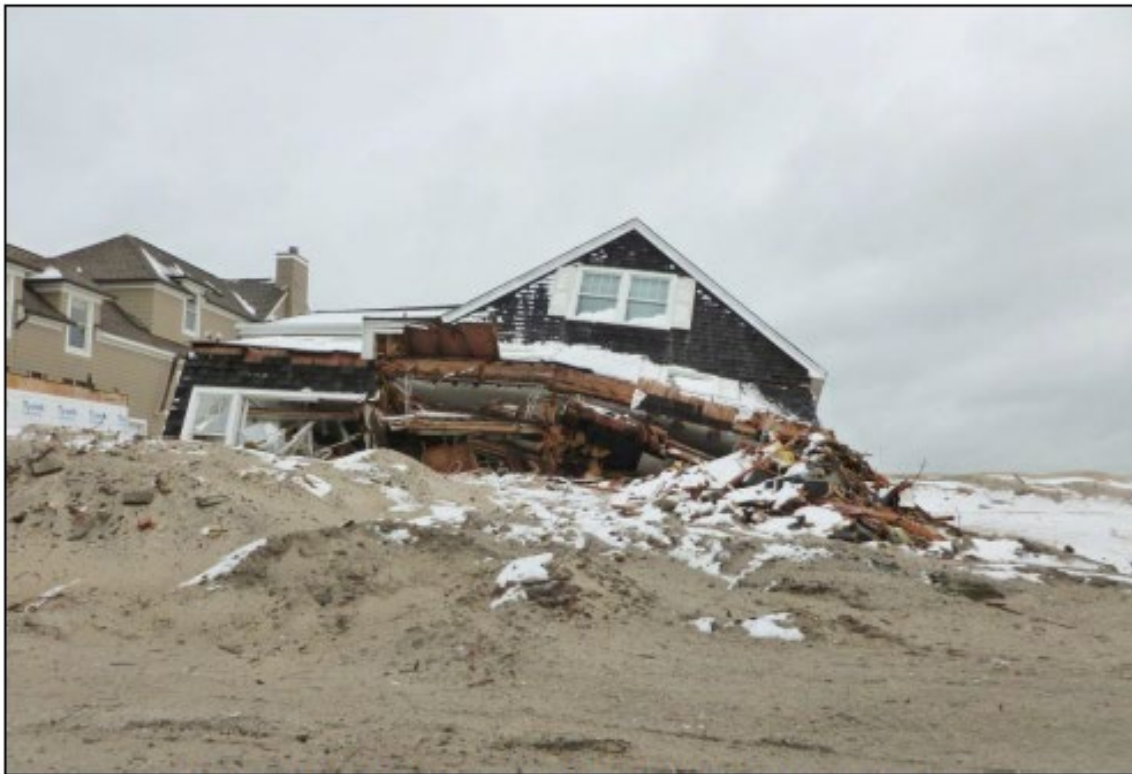
Image #2: The above example photo illustrates pancaking.
