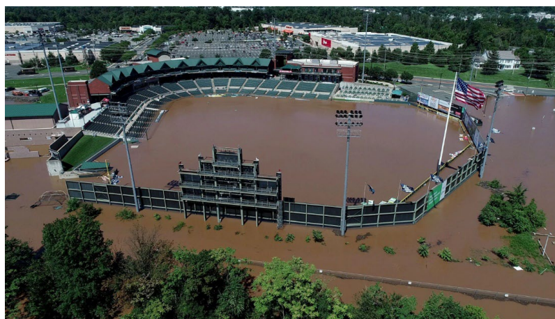
Figure 8: TD Bank Ballpark Flooded With Water Due to Hurricane Ida
