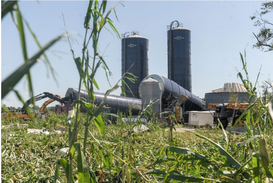
Figure 10: Tornado Damage at Wellcrest Farms in Mullica Hill, NJ, September 2, 2021
