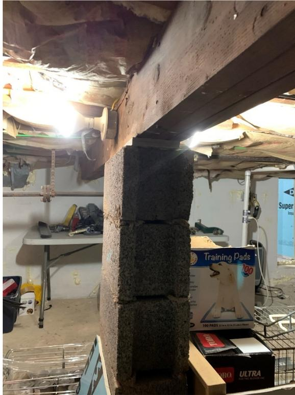
**Photo 7. Girder with CMU Pedestal in East Crawl Space (Looking West)**
