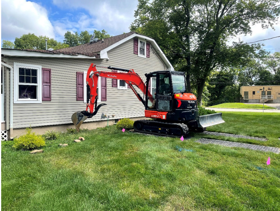
Photo 13. Test Pit TP-1 Location (South Wall of Building – Crawl Space)
