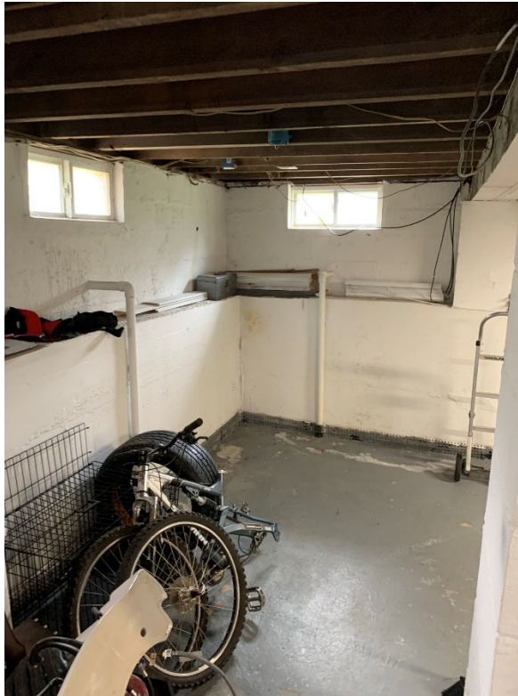
Photo 4. Basement CMU/Concrete Wall and Timber Subfloor (Southeast Corner)
