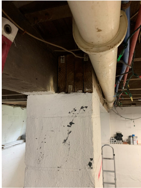
Photo 5. Front Basement Girder with Additional (4) 2x8 Beams for Southeast Corner
