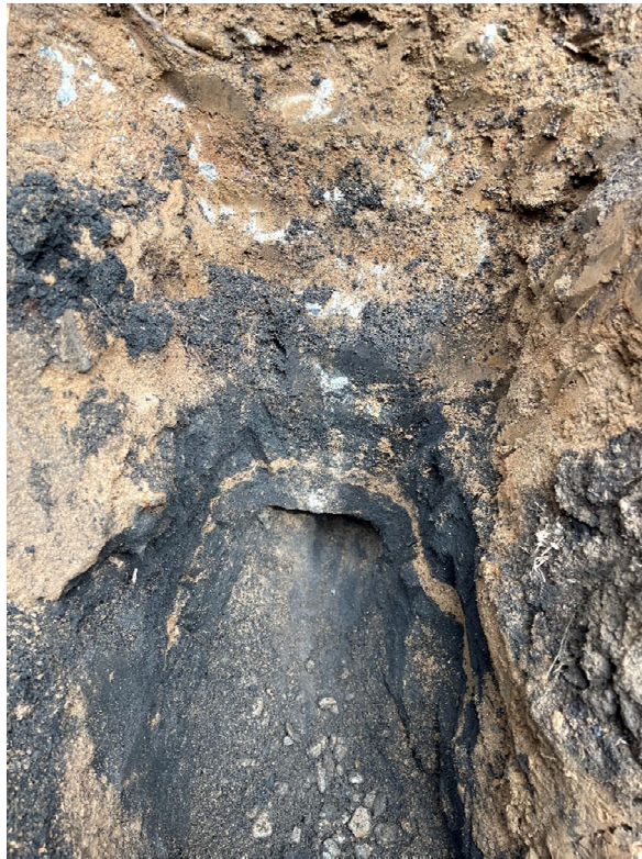
Photo 14. Test Pit TP-1 Foundation Conditions
