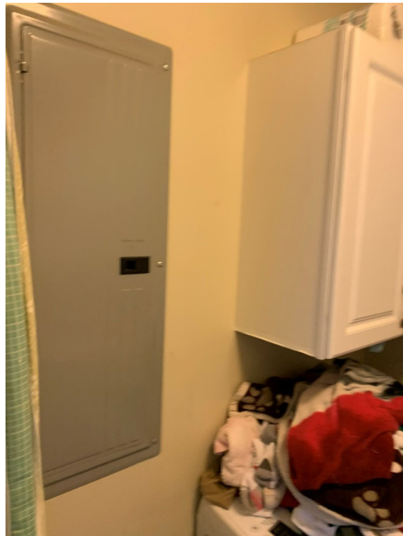
Photo 12. Electrical Panel in First Floor Laundry Room
