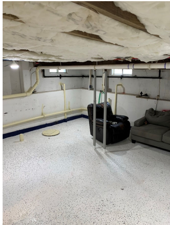
Photo 8. Front Basement Northeast Corner
