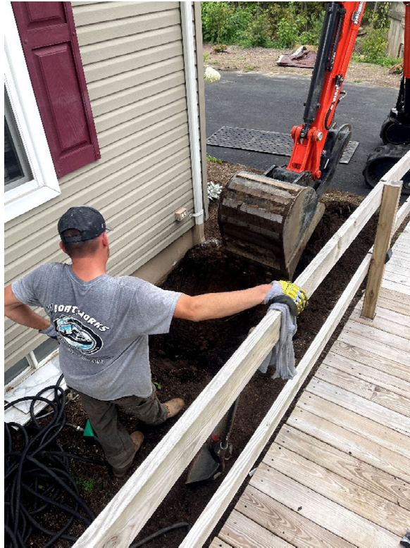
Photo 15. Test Pit TP-2 Location (Front Wall of Building – Northeast Corner)
