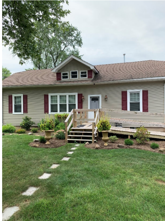
Photo 1. 140 Little Falls Road (Front of Building)
