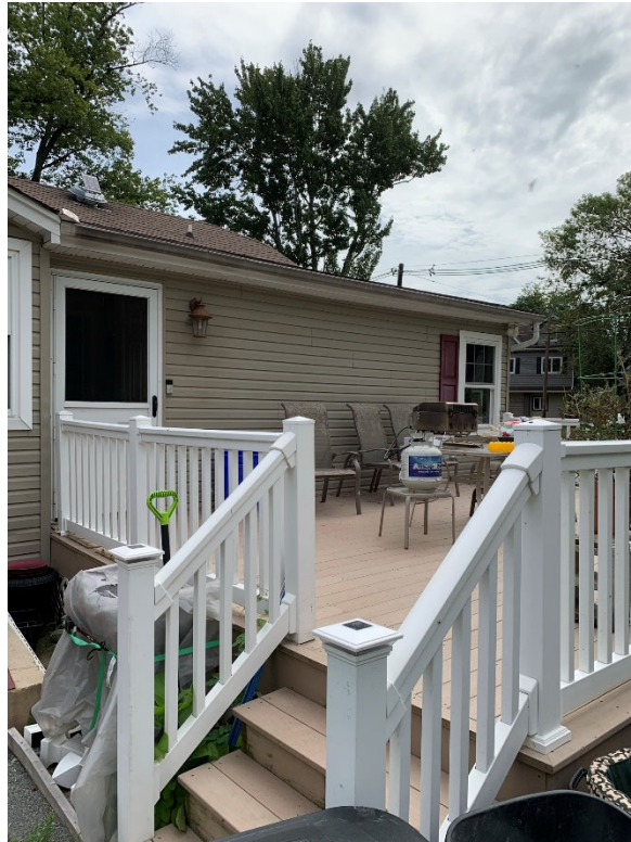
Photo 3. 140 Little Falls Road (Rear Addition with Timber Deck)
