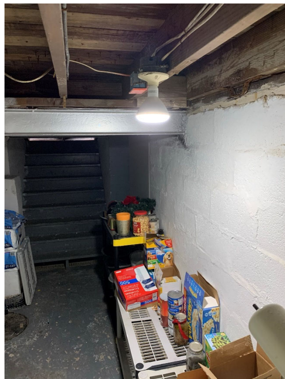
Photo 10. Backyard Access Basement Room (Looking at Building Rear)
