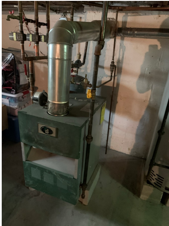
Photo 7. Boiler on CMU Blocks (Basement)
