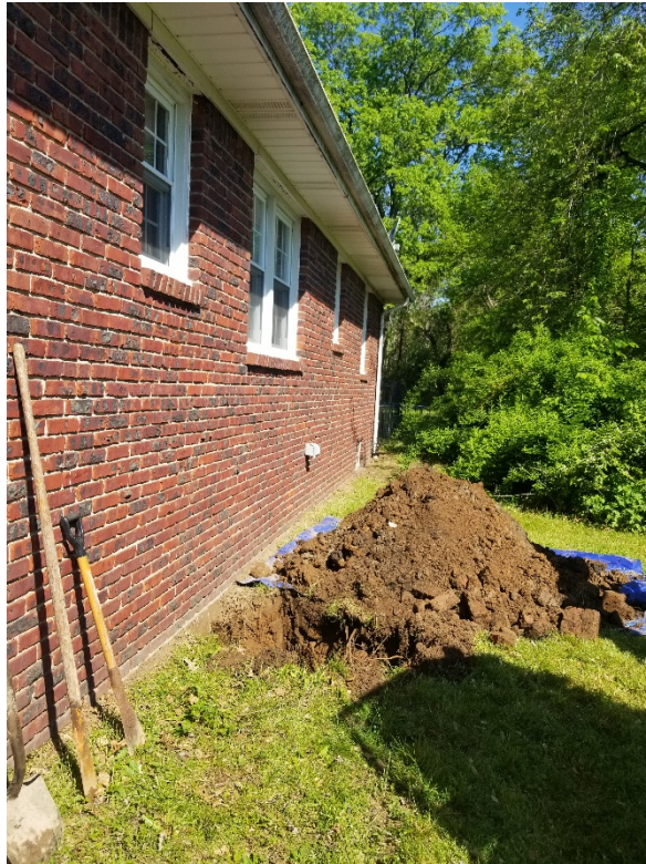
Photo 15. Test Pit TP-2 Location (East Wall of Building – Crawl Space)
