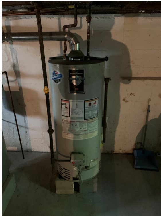
Photo 6. Water Heater on CMU Blocks (Basement)
