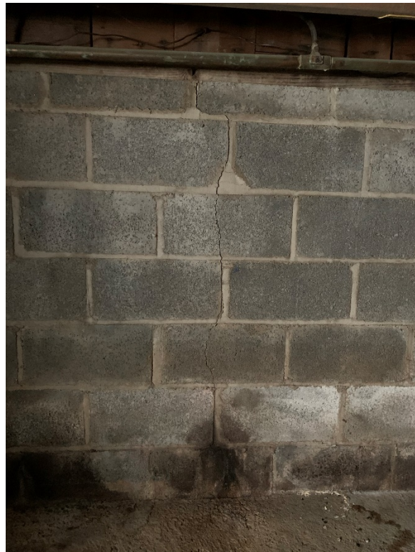
Photo 10. Vertical Crack in South Crawl Space Wall (Typical for Two)
