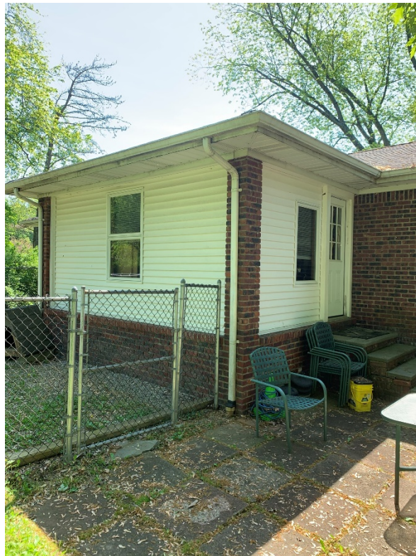
Photo 3. 1 Matt Drive (Rear Addition)
