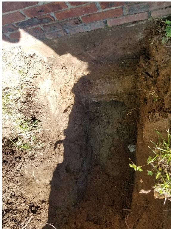
Photo 14. Test Pit TP-1 Foundation Conditions
