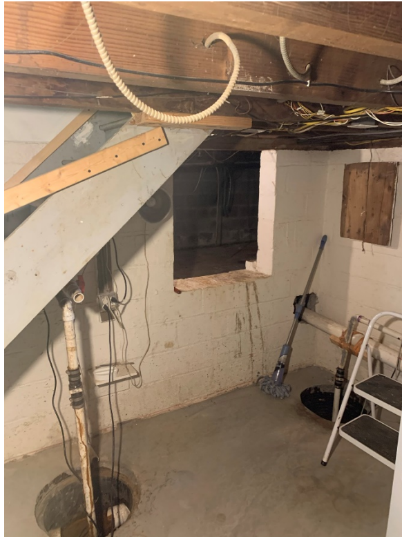
Photo 5. Basement Sump Pumps and Opening to Crawl Space
