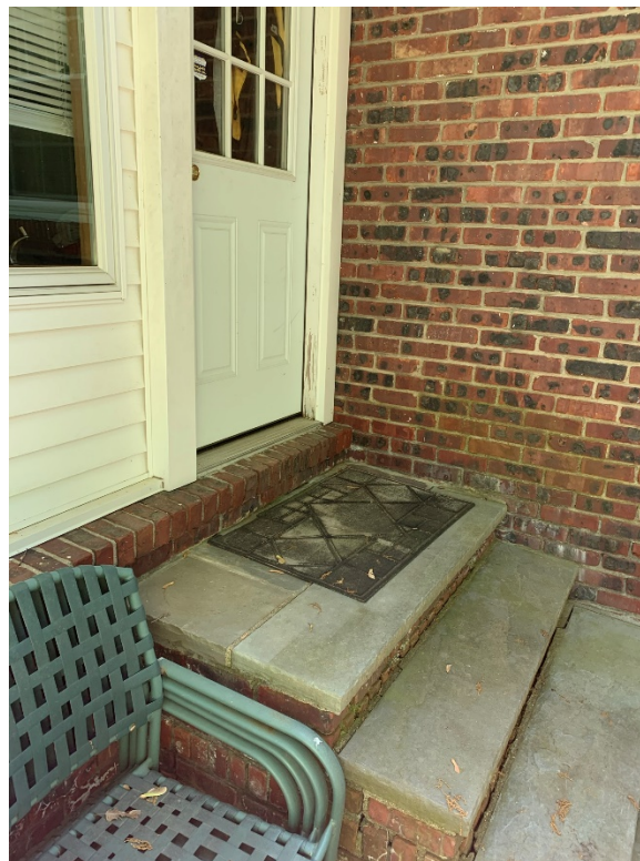
Photo 12. Stairs to Rear Addition Entrance Door
