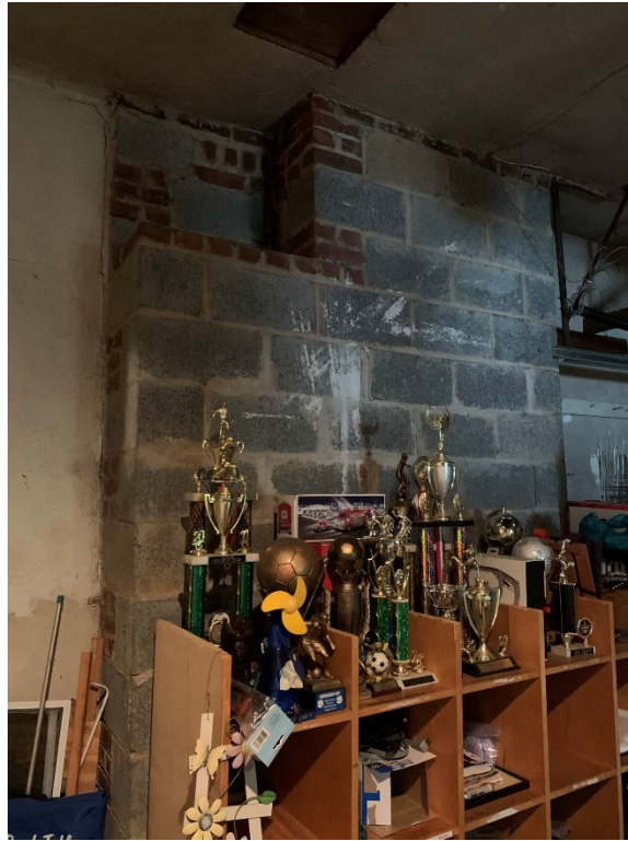
Photo 11. Chimney (East Garage Wall)
