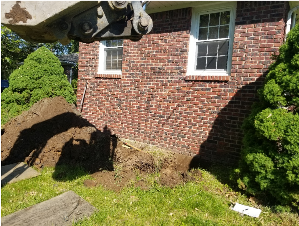
Photo 13. Test Pit TP-1 Location (Front of Building – Crawl Space)
