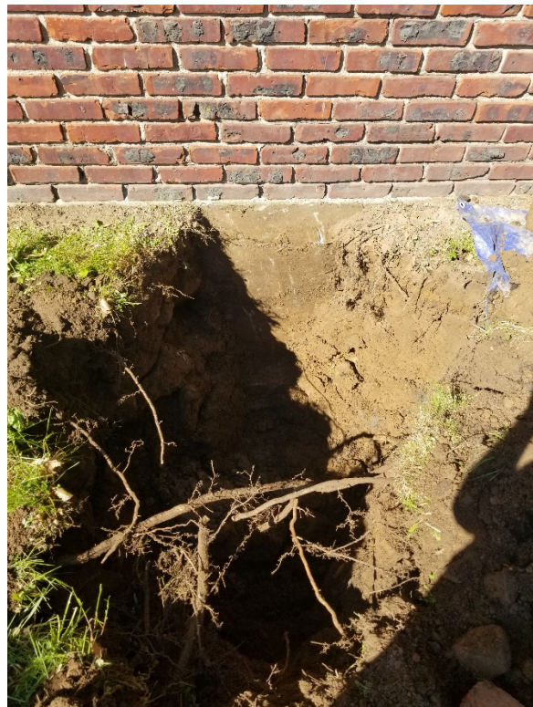
Photo 16. Test Pit TP-2 Foundation Conditions
