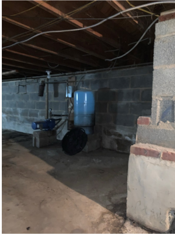
Photo 9. Water Storage Tank and Pump (West Edge of Crawl Space)
