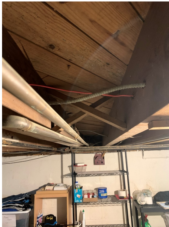
Photo 4. Basement CMU Wall and Timber Subfloor
