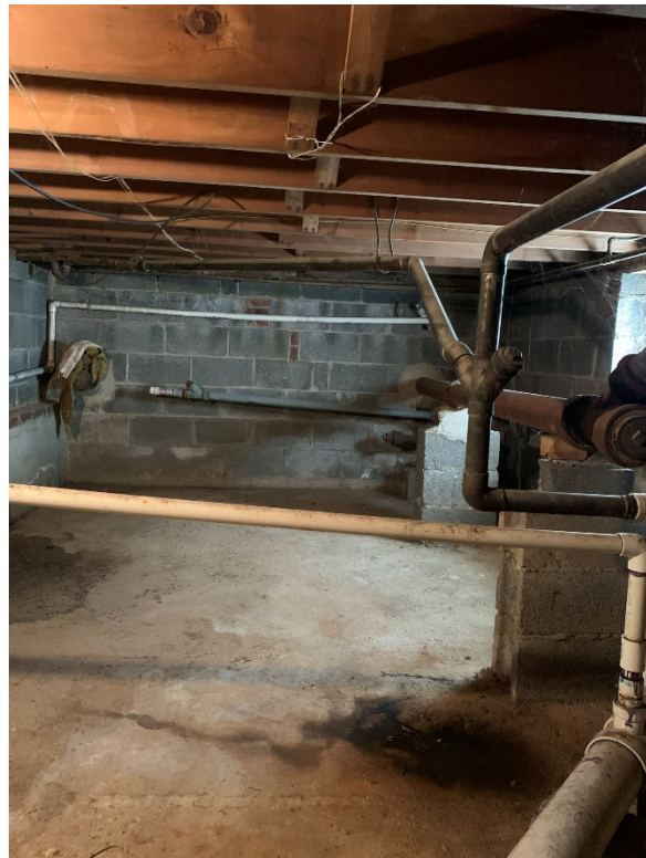
Photo 8. Crawl Space CMU Walls and Timber Subfloor (Looking North)
