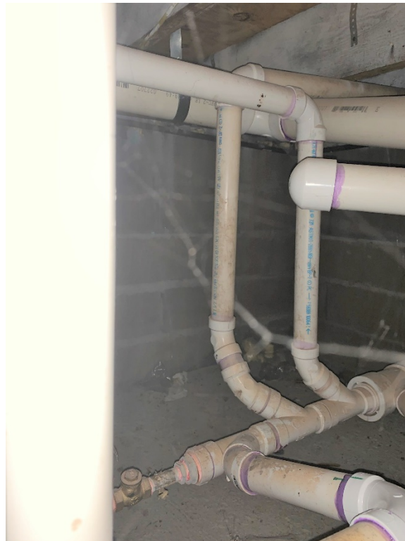
Photo 6. Southeast Crawl Space
