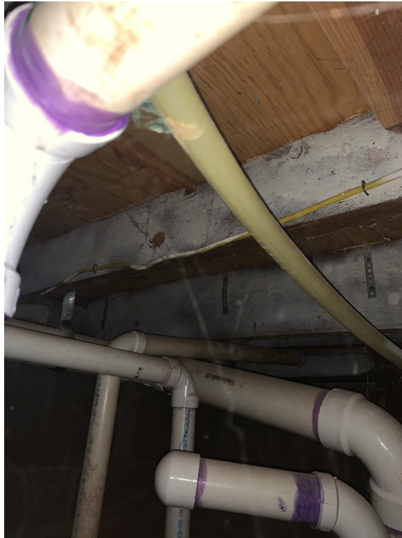
Photo 7. Floor Joist in Southeast Crawl Space
