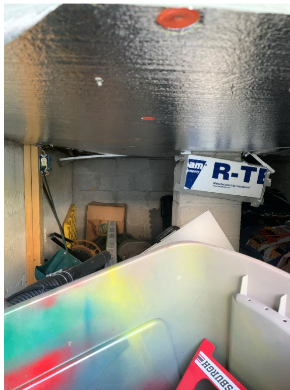
Photo 10. Front Crawl Space CMU Walls and Pedestal (Looking South)
