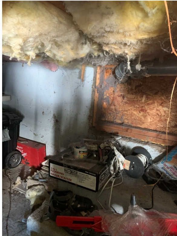
Photo 9. Concrete Steps and Boarded Up Opening in West Wall of Northeast Crawl Space
