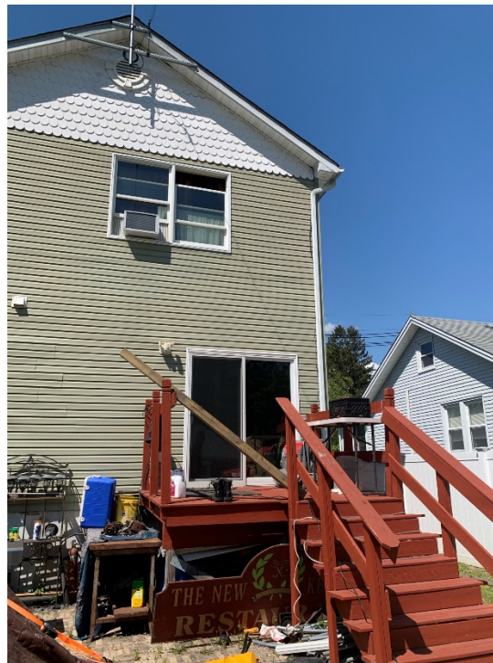
Photo 2. 38 Clinton Road (Rear of Building)
