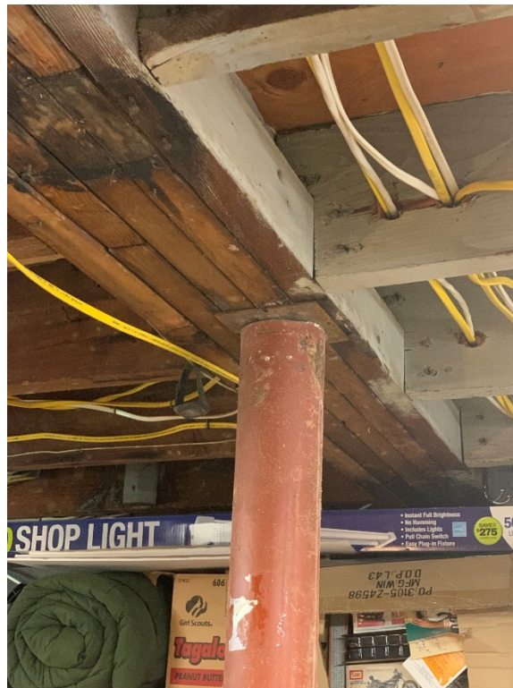
Photo 4. Steel Post Support for Basement Girder (Typ.)
