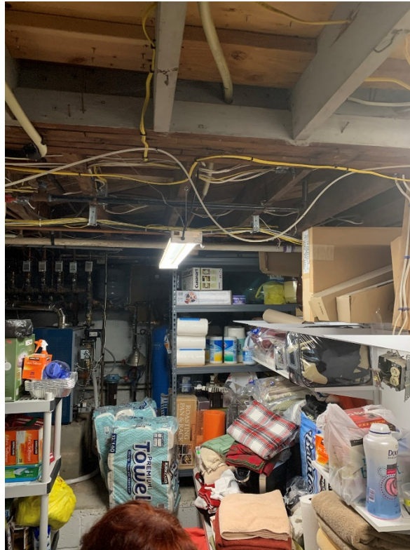
Photo 3. Floor Joists and Girder in Basement
