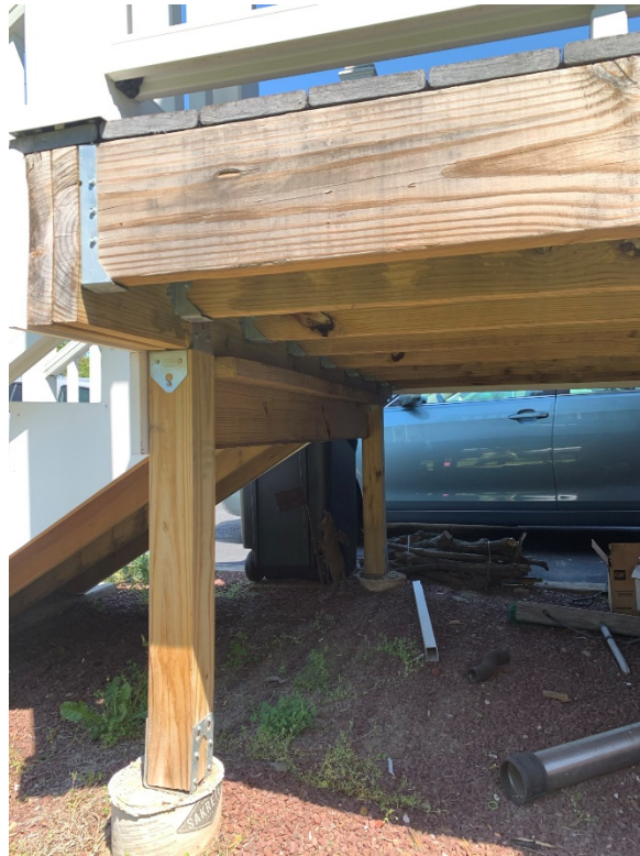
Photo 11. Front Entrance Stairs Frame and Supports
