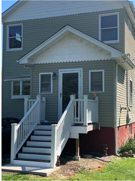
Photo 1. 38 Clinton Road (Front of Building)
