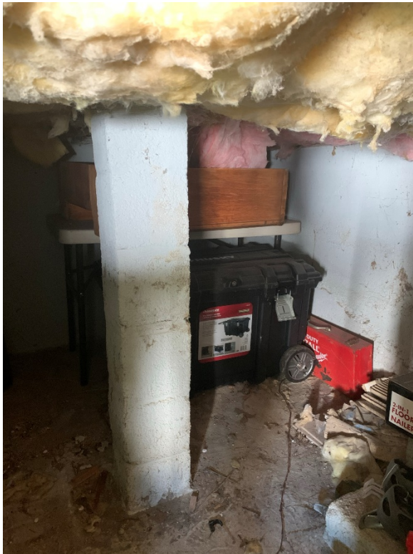
Photo 8. Northeast Crawl Space CMU Pedestal (Looking South)
