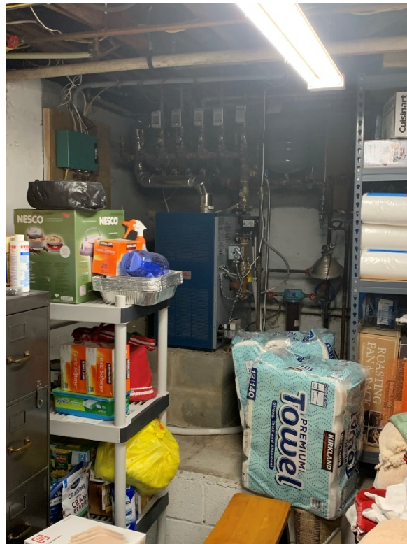
Photo 5. Boiler and Water in Basement (Southeast Corner)
