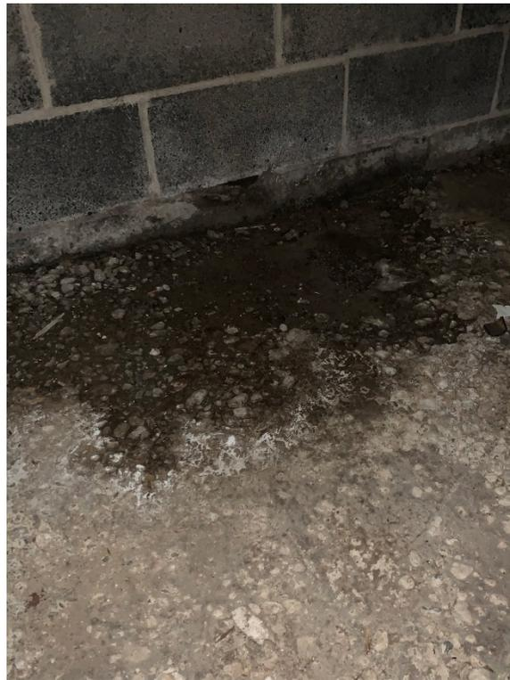
**Photo 6. Water Infiltration in Crawl Space (North Wall)**
