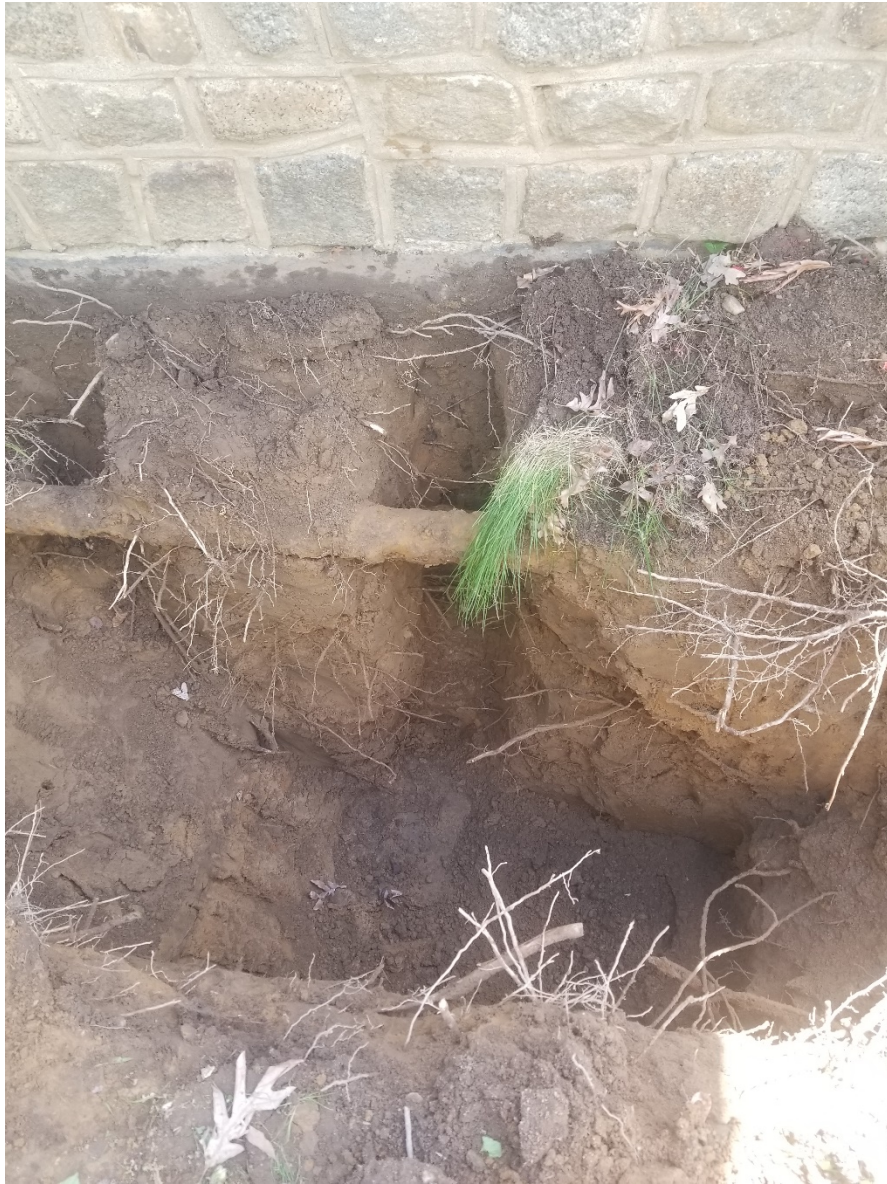
Photo 13. Test Pit TP-2 Conditions
