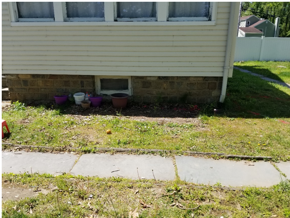
Photo 12. Test Pit TP-2 Location (North Wall of Building – Basement)
