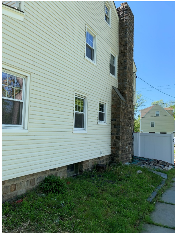
Photo 3. West Wall of Building with Chimney
