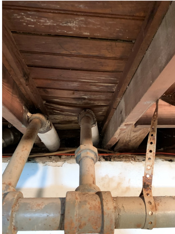
Photo 9. Typical First Floor Subfloor in Basement
