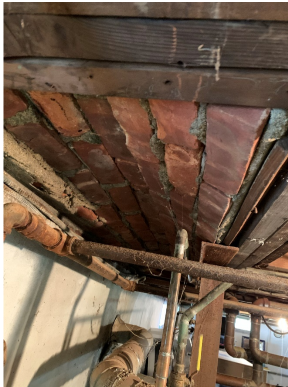
Photo 4. Bottom of Chimney in Basement (Along West Wall – Looking North)
