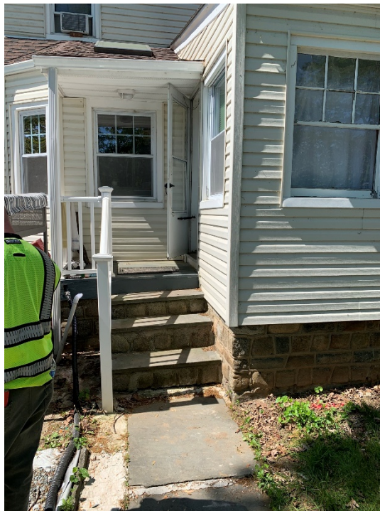
Photo 2. 47 Riveredge Drive (Rear of Building)
