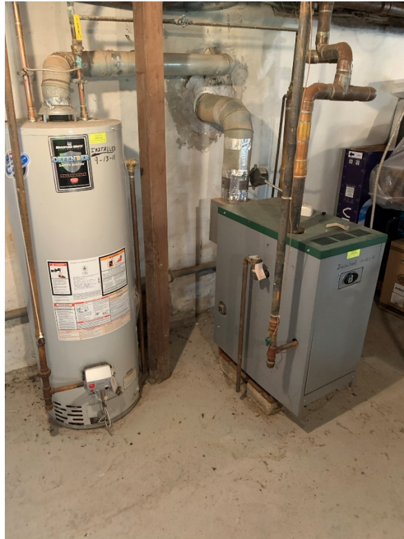
Photo 7. Water Heater & Boiler in Basement (West Wall)
