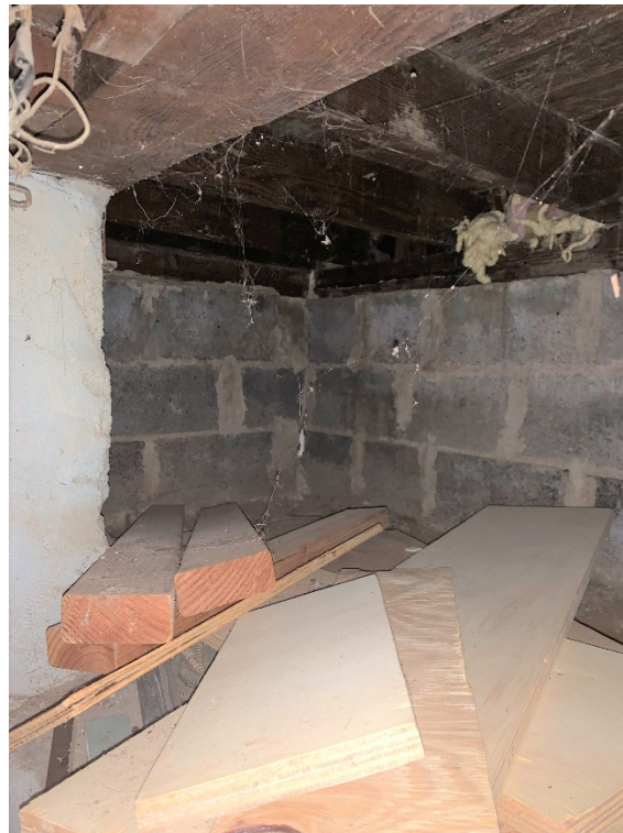
Photo 10. Front Crawl Space with CMU Walls (Looking South)
