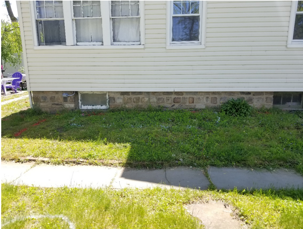
Photo 11. Test Pit TP-1 Location (West Wall of Building – Basement)
