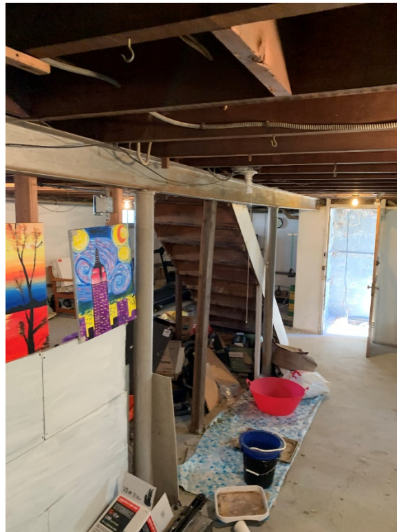
Photo 8. Steel Girder Supporting First Floor Joists (Looking North)
