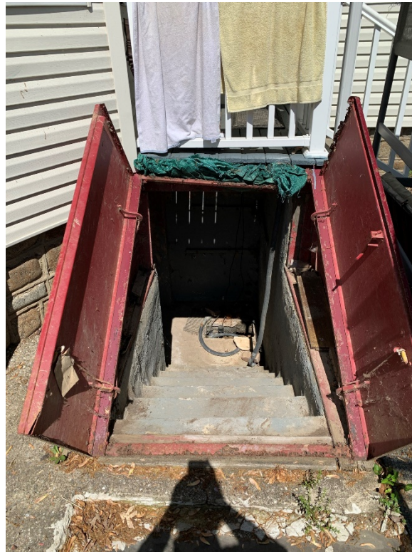
Photo 5. Rear Stairs to Basement
