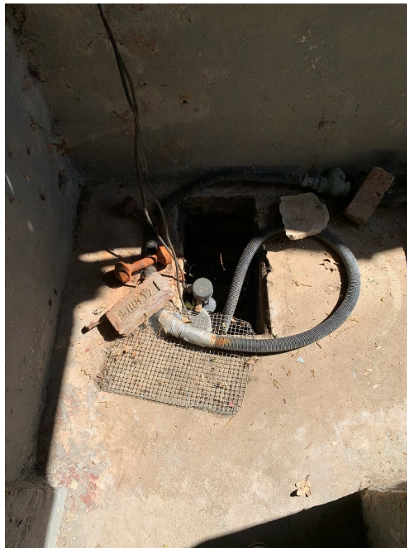
Photo 6. Sump Pit in Rear Stair Enclosure
