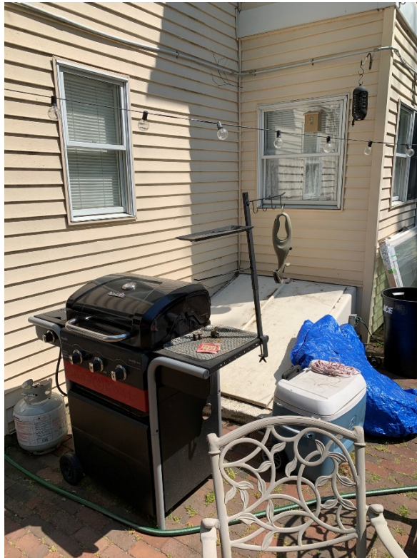
Photo 3. 90 Pier Lane (Rear of Building – East Side)
