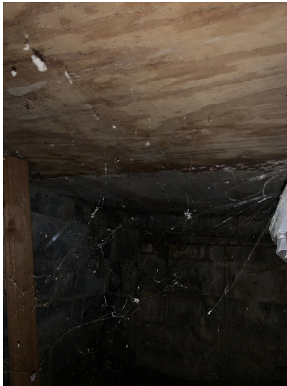
Photo 6. Rear Offshoot of Rear Basement Space (Looking South)
