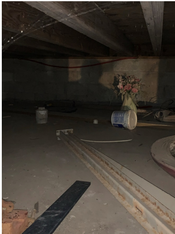
Photo 8. Crawl Space Area (Looking West)
