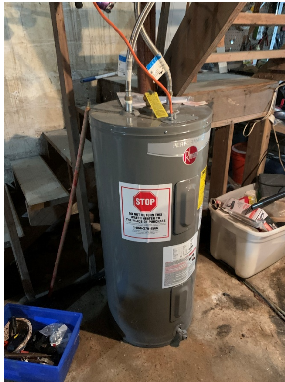
Photo 10. Water Heater in Basement
