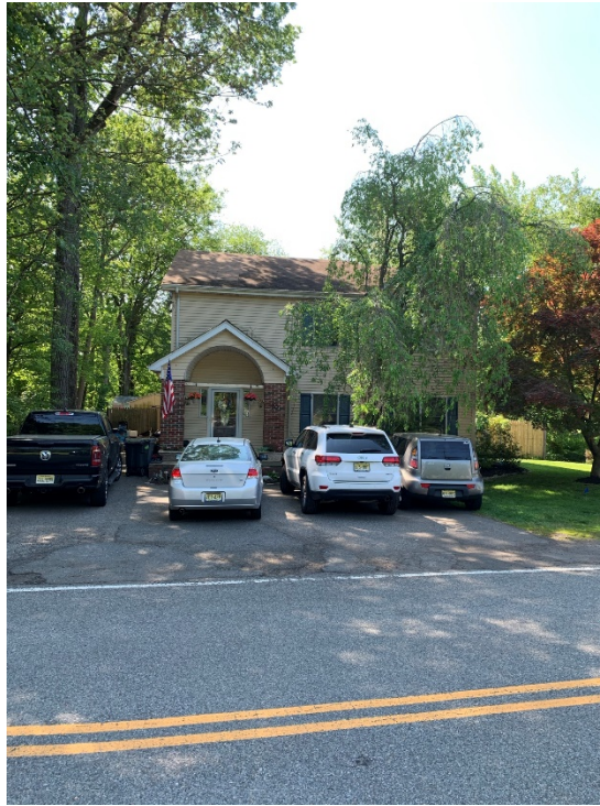
Photo 1. 90 Pier Lane (Front of Building)
