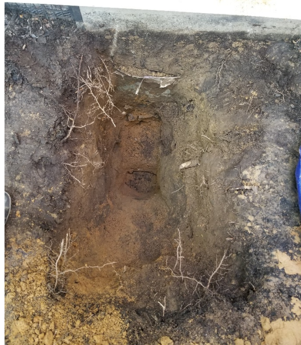
Photo 14. Test Pit TP-1 Foundation Conditions
