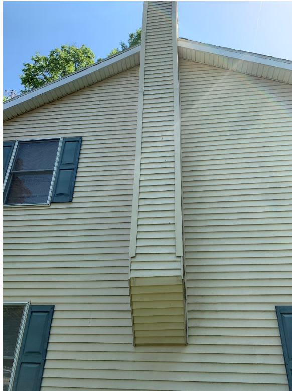
Photo 11. Chimney Off West Wall of Building
