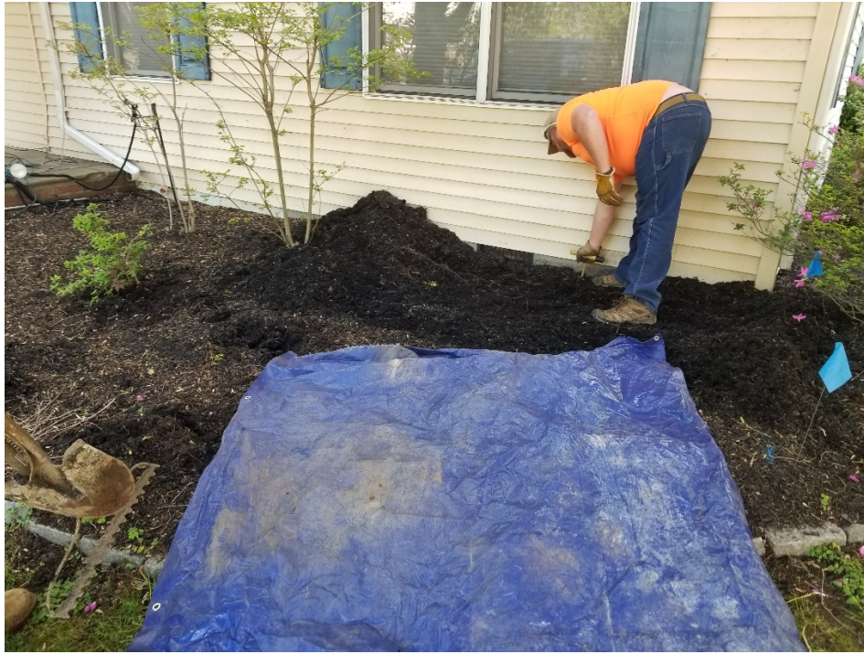
Photo 13. Test Pit TP-1 Location (Northwest Corner of Building – Crawl Space)
