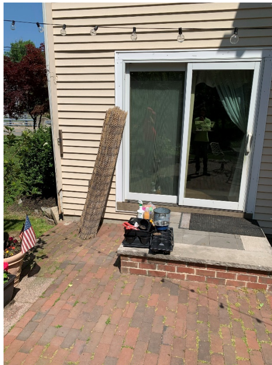
Photo 2. 90 Pier Lane (Rear of Building - West Addition)
