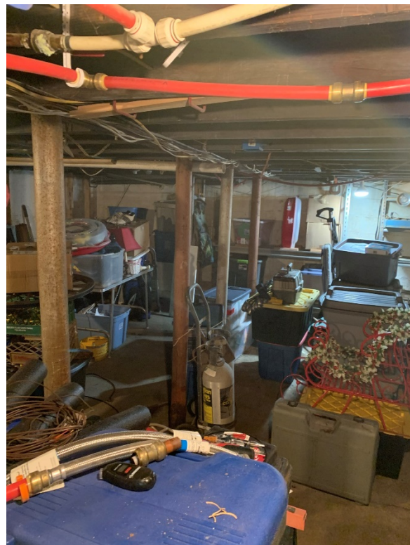
Photo 4. First-Floor Girder & Steel Support Posts (Looking North)
