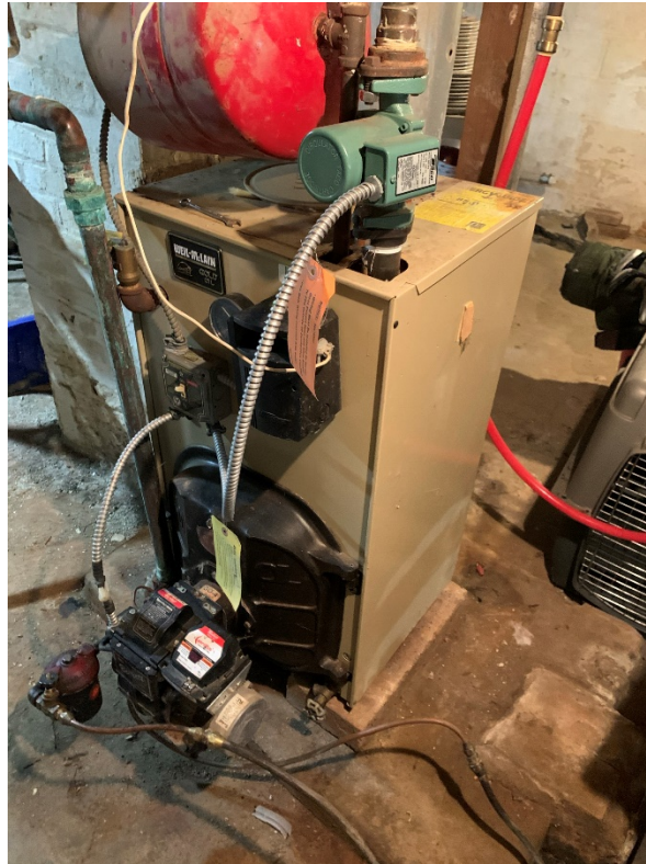
Photo 9. Boiler in Basement
