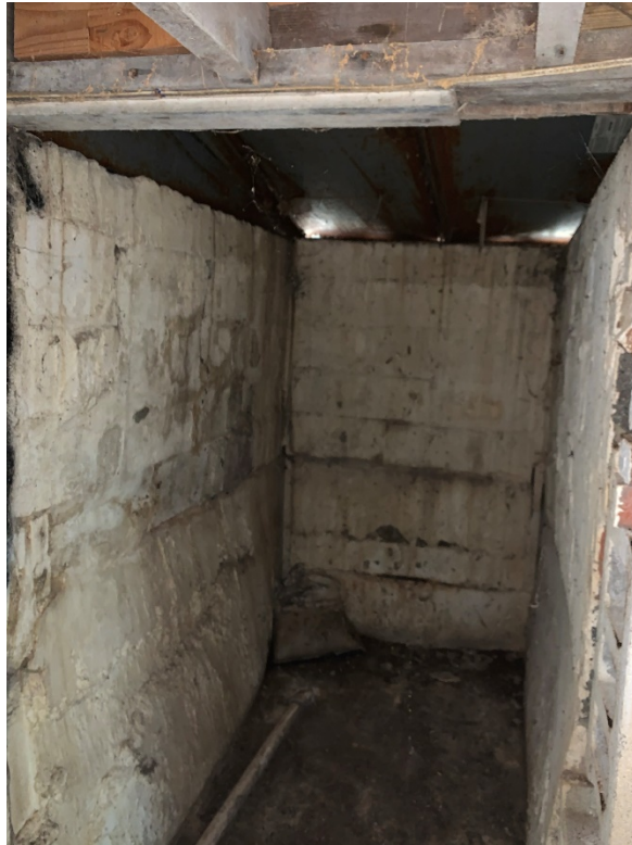
Photo 5. Rear Area of Basement (Looking West)
