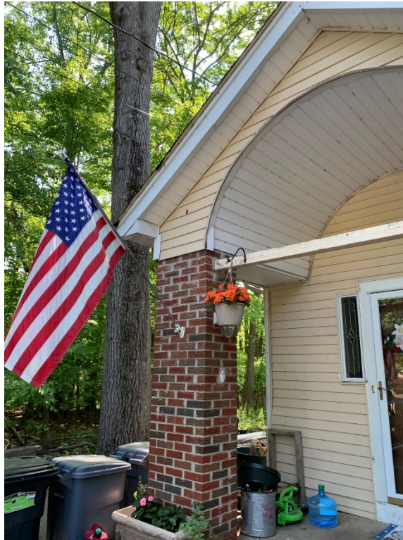
Photo 12. Entrance Archway with Brick-Encased Columns
