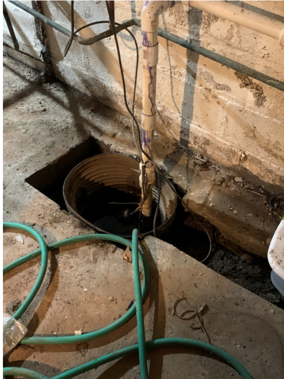
Photo 7. Sump Pit in Unfinished Trench (Southwest Corner of Basement)
