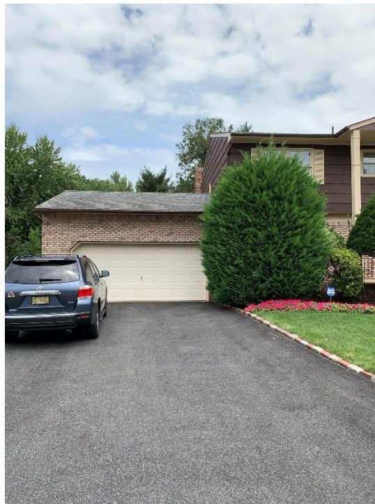
Photo 2. 93 Glenroy Road East (Front of Attached Garage)
