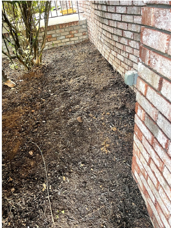
Photo 13. Test Pit TP-1 Location (Front of Building – Basement, Southwest Corner)
