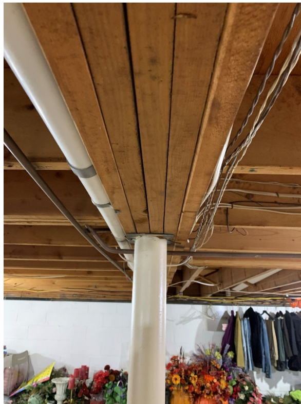
Photo 6. Timber Girder with Steel Post Column (Typical)
