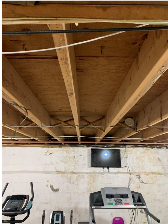
Photo 7. First Floor Timber Floor Joists (Typical)
