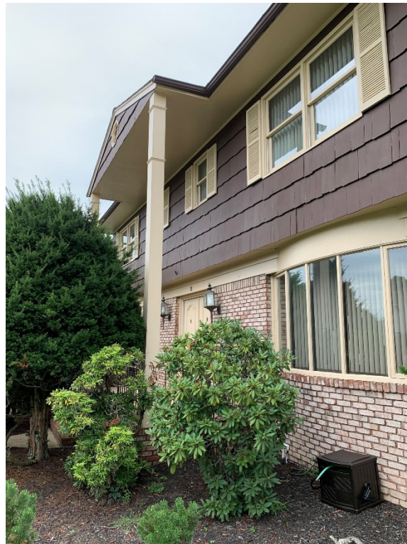
Photo 12. Roof Overhang with Column Supports on Front Porch
