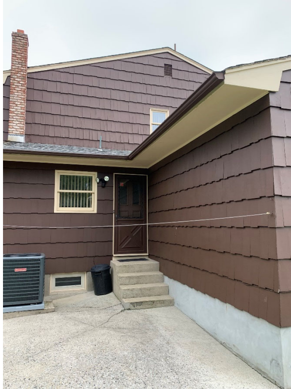
Photo 3. 93 Glenroy Road East (Rear of Building, West Side)
