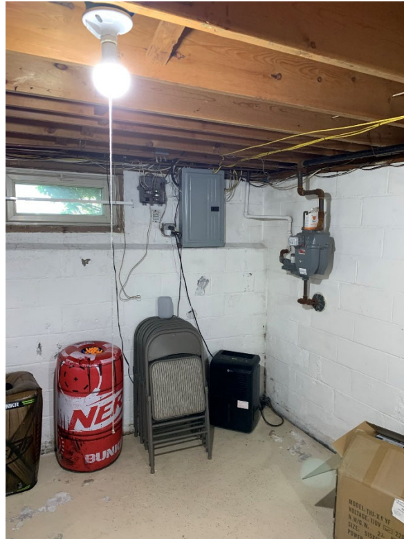
Photo 9. Gas Meter & Electrical Panel in Basement (Looking South)
