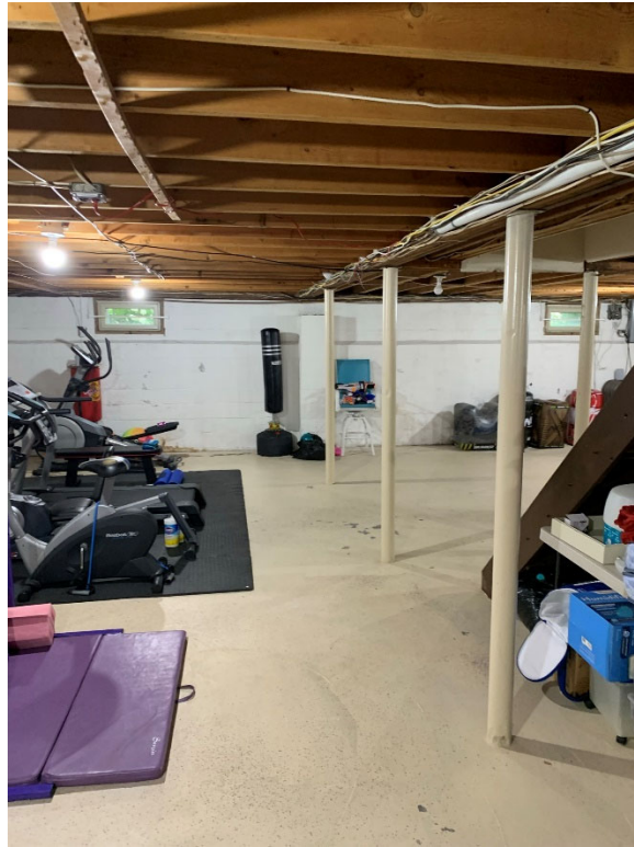
Photo 5. Basement CMU Walls and First Floor Subfloor (Looking Southeast)
