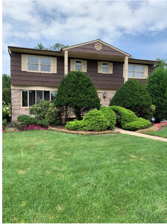
Photo 1. 93 Glenroy Road East (Front of Building)
