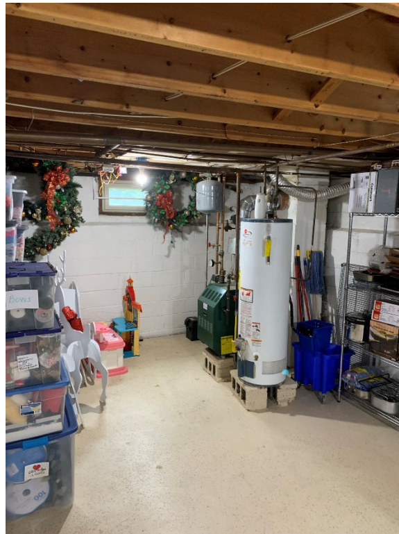
Photo 8. Boiler & Hot Water Heater in Basement (Looking North)
