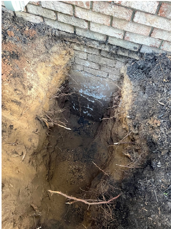
Photo 14. Test Pit TP-1 Foundation Wall Conditions
