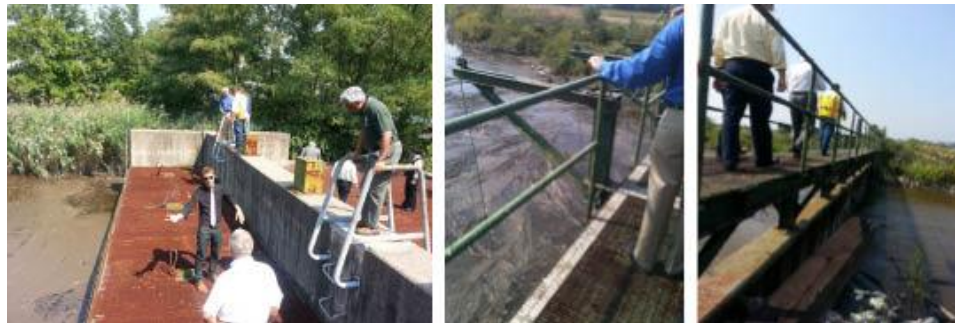
Figure 3-1: Physical Inspection of Existing Risk Reduction Infrastructure. Teams assigned by the New Jersey Department of Environmental Protection have endeavored to catalogue Superstorm Sandy’s impact on berms, tidal gates, and other existing risk-reduction infrastructure. Physical inspection is a key part of the State’s assessment of the current condition of measures to identify necessary repairs as well as opportunities to enhance existing measures to address future extreme weather events and maximize federal investment.
