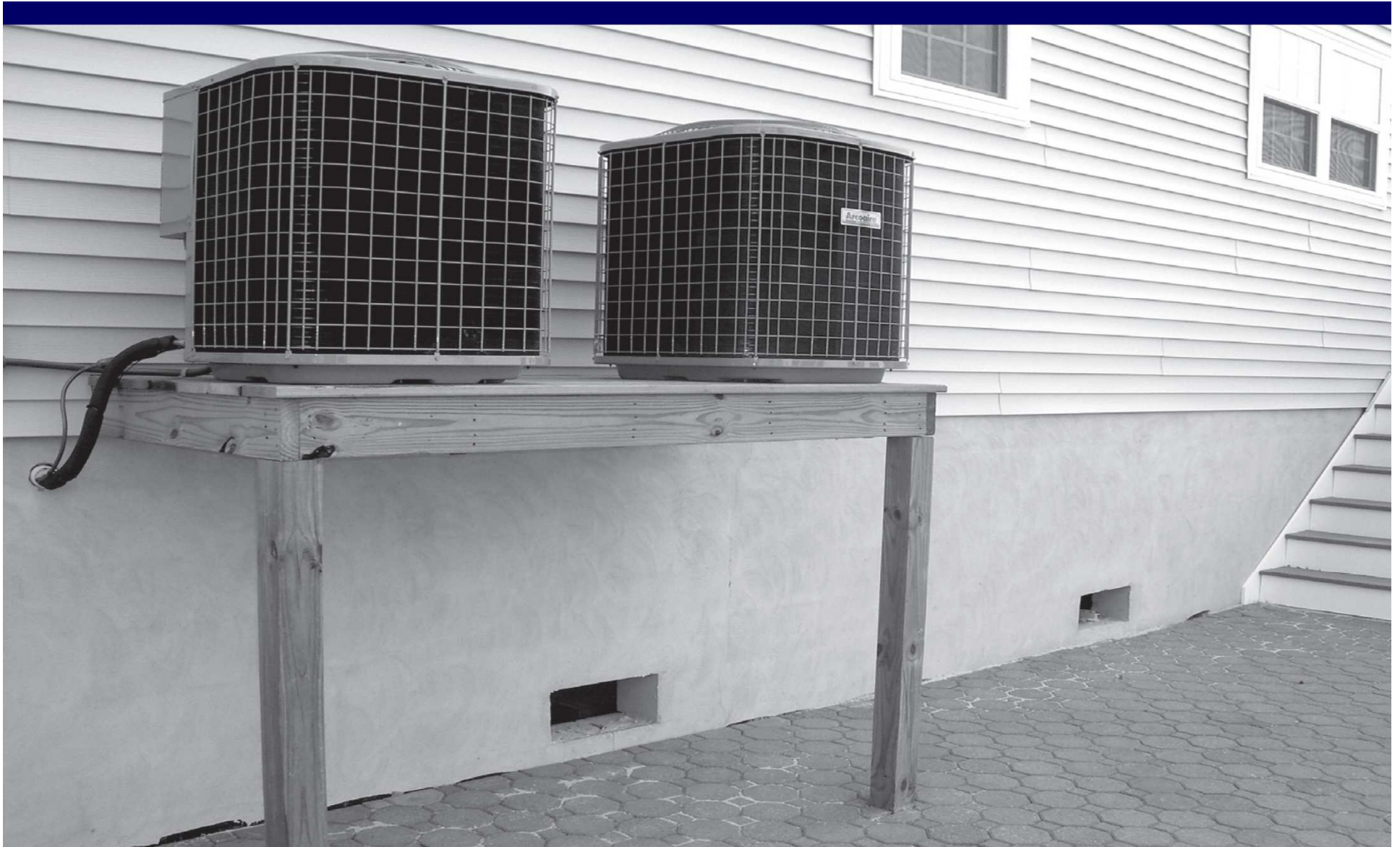
Foundation wall with omitted blocks as flood openings (insect screen not visible)
