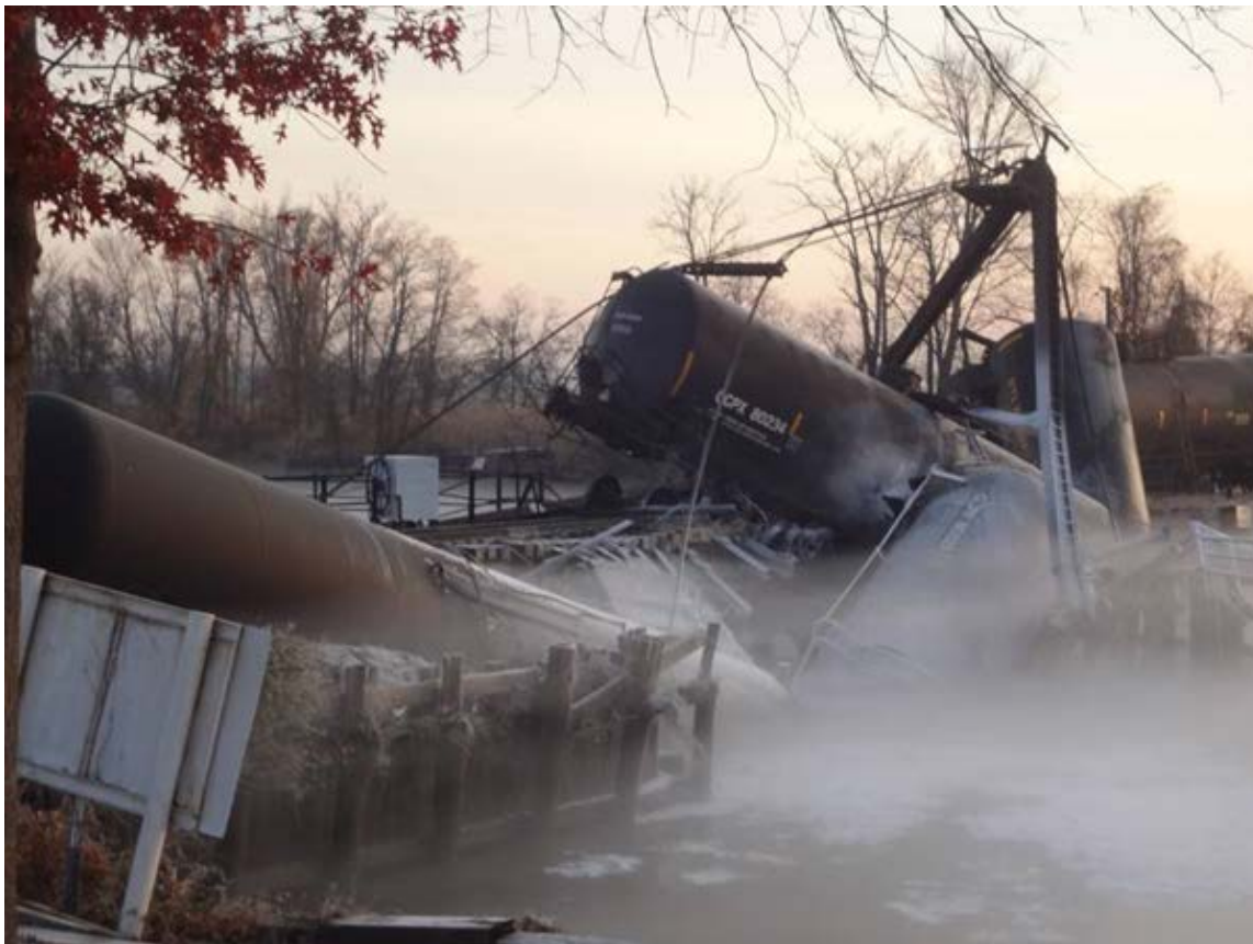
Figure 10. The breached tank car leaning off the bridge and the vinyl chloride vapor cloud. (Photograph provided by a private citizen)
