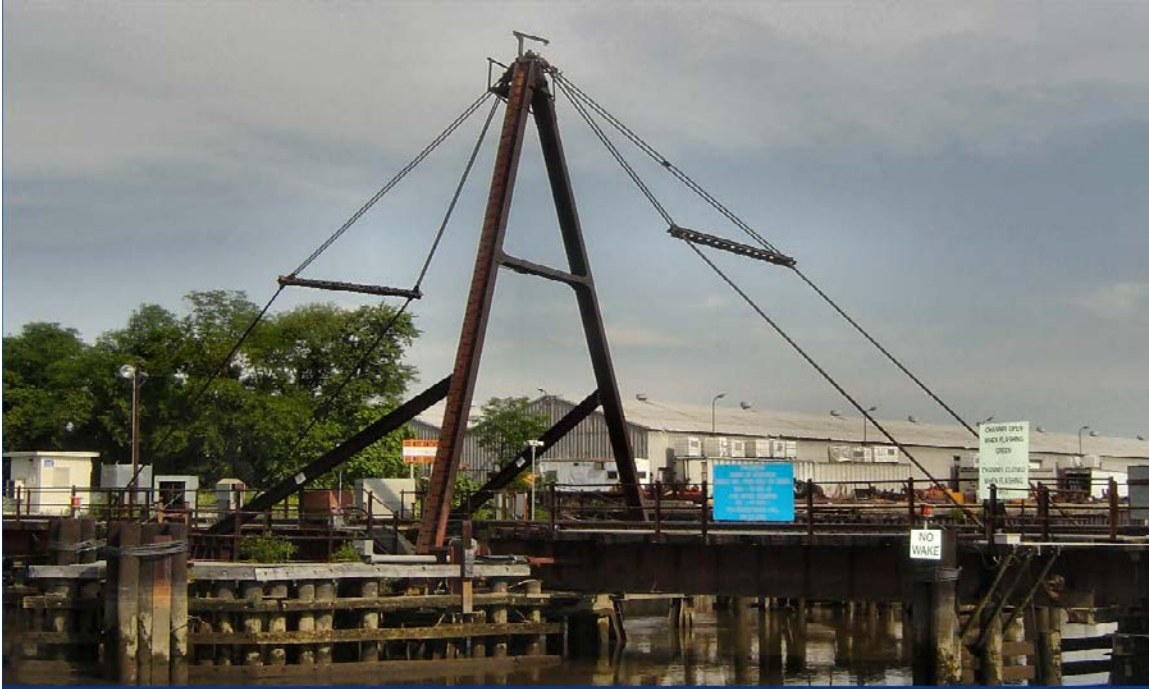
Figure 4. Preaccident photograph of the Paulsboro moveable bridge. (Photograph provided by Conrail.)
