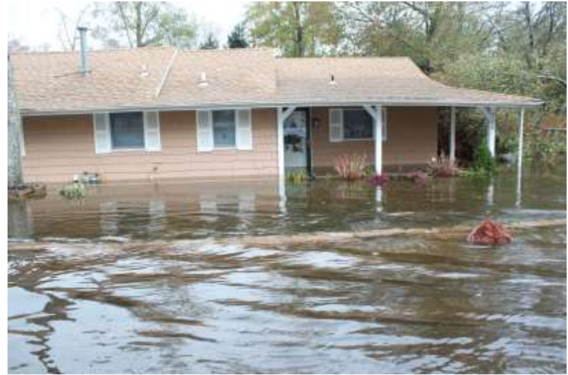
Figure 3: Damage to Residential Property (2 of 2)
