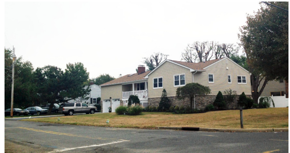
Residence with living space above the flood elevation
