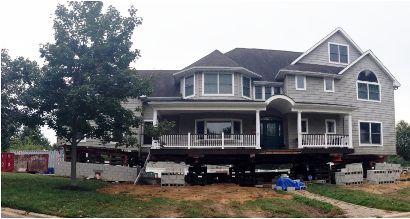
Residence in the process of being lifted above the flood elevation
