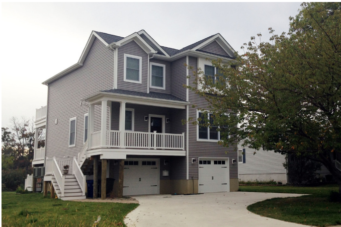
Residence with living space above the flood elevation
