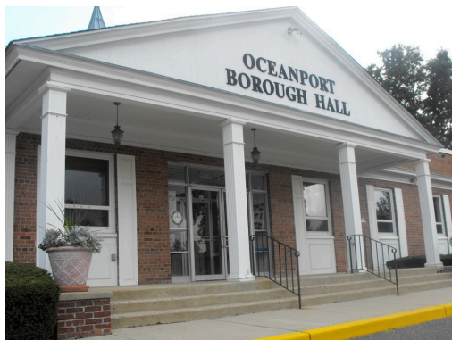
Existing Municipal Building that suffered substantial damage from Superstorm Sandy
