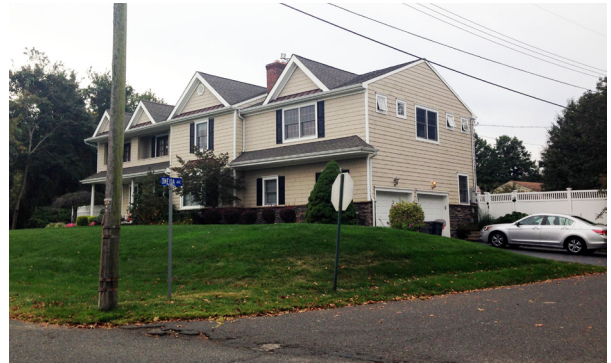
Residence whose ground elevation was raised in response to flooding
