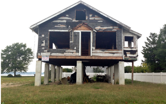
Residence that suffered substantial damage during Superstorm Sandy
