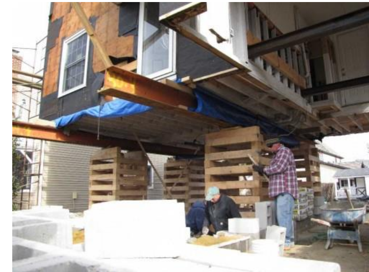
Figure 4: A Rumson Home is Elevated.
