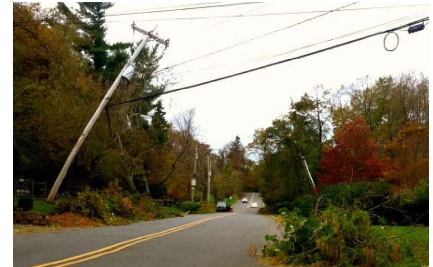
Figure 3: Wind Damage in Rumson Borough
