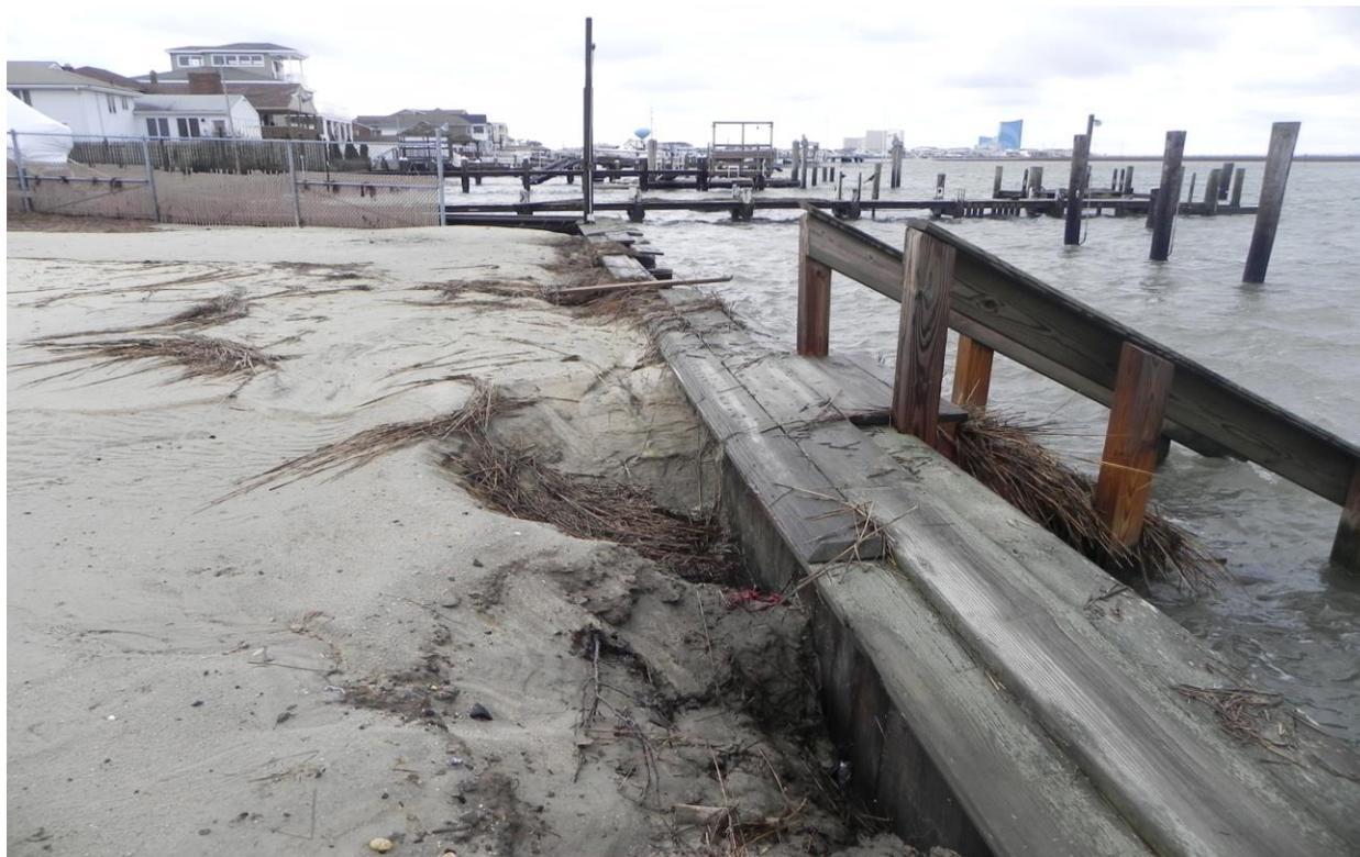
**Figure 30 – City Dock Damage Caused by Superstorm Sandy**
