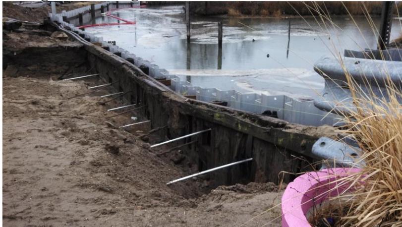
Figure 8: Damage to the Waackaack Creek Bulkhead (2)
