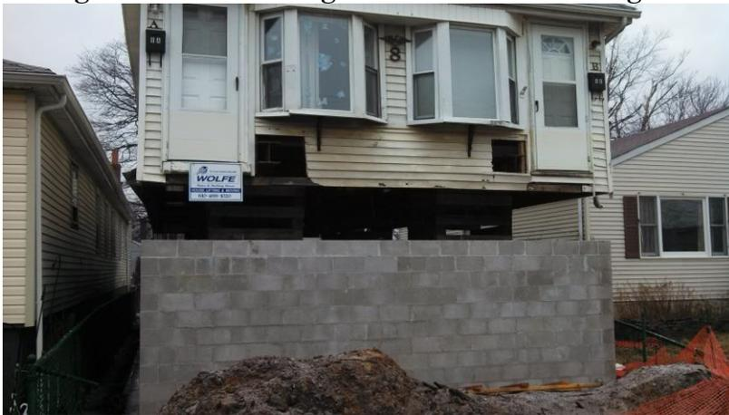
**Figure 31: A Keansburg Home Elevation in Progress (2)**
