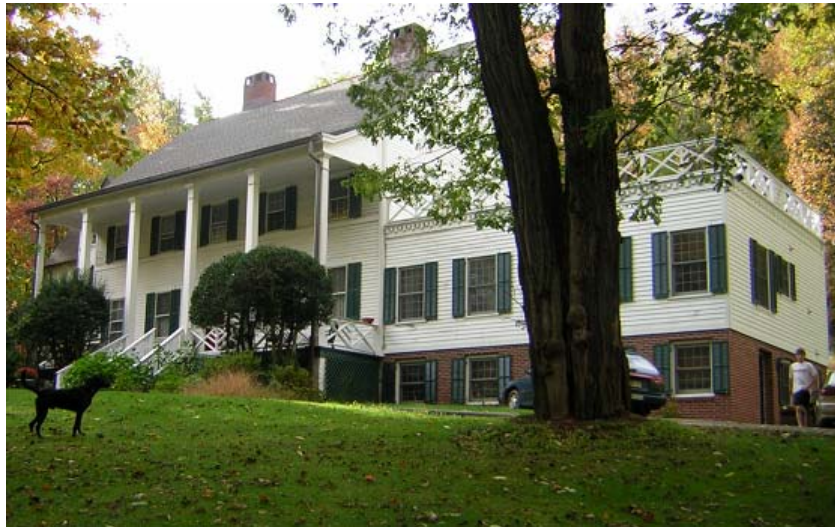
Figure 77: Peter Kemble House Site Source: Photograph by the Author
