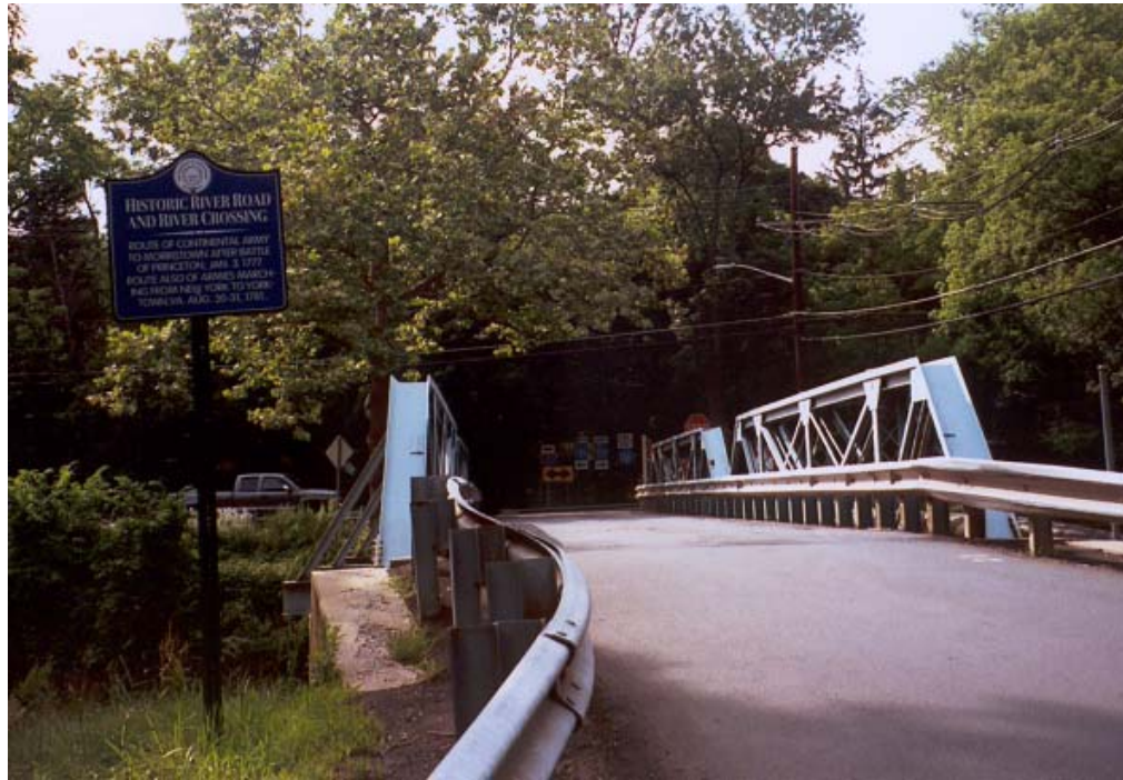
Figure 95: Bridge over the Millstone River Source: Photograph by the Author
