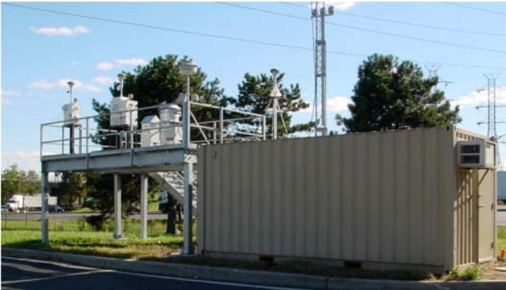
Air Monitoring Shelter
