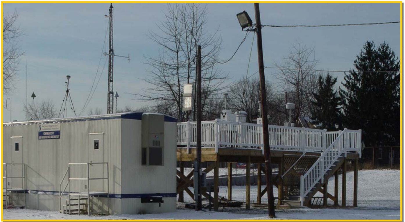
Comprehensive Air Monitoring Station – Camden, New Jersey
