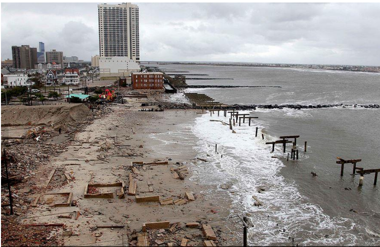
Image 2: Superstorm Sandy Damage of the AC Boardwalk (LA Times)
