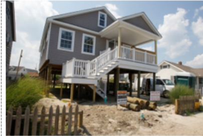
Figure X. Elevated home in Manasquan, Source: Patti Sapone, The Star-Ledger
