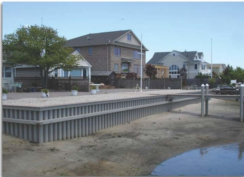
Bulkheads, such as the structure pictured above, are built to prevent erosion caused by high tide flooding.
