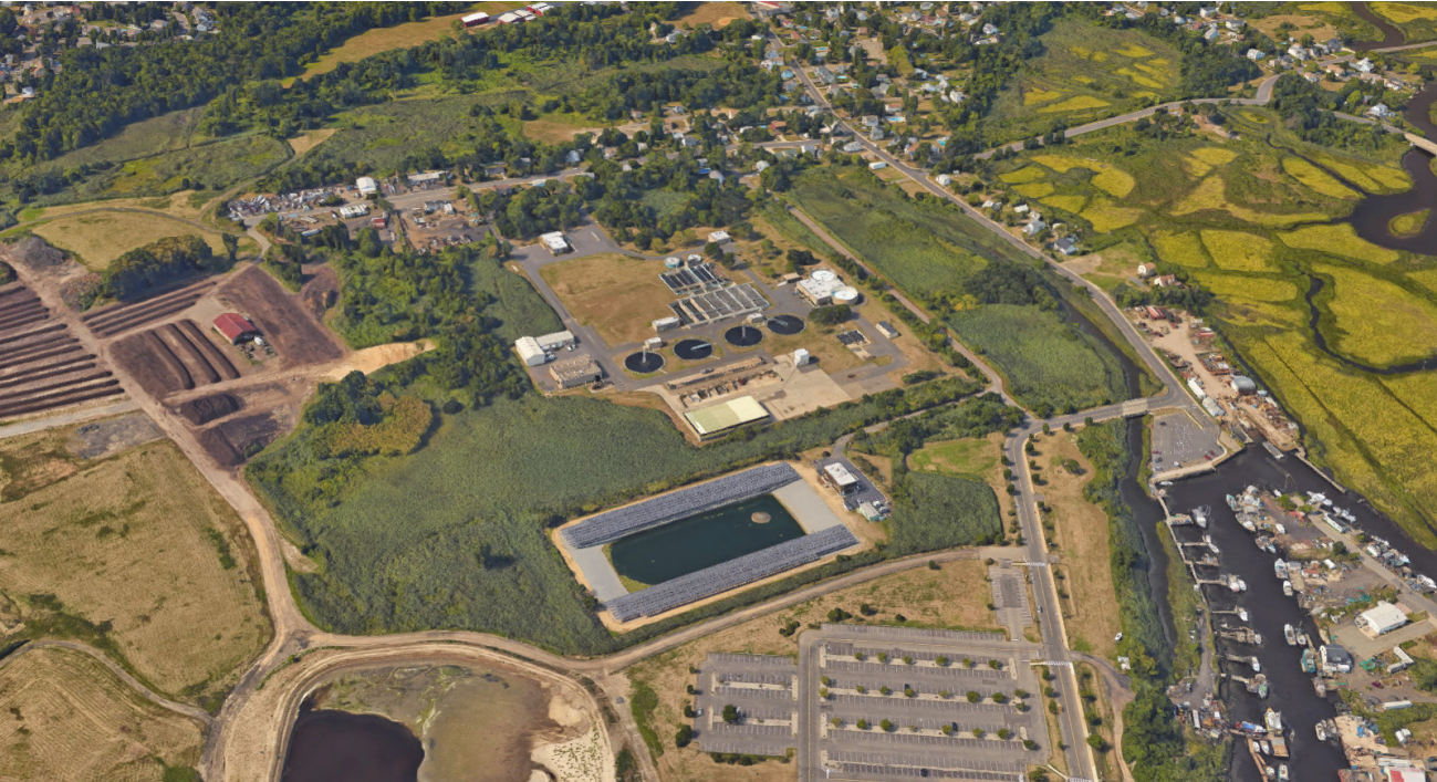
Middletown Township Sewage Authority Treatment Plant, 2020
