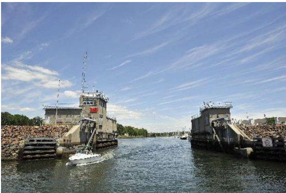
Stamford hurricane barrier, Stamford, CT
