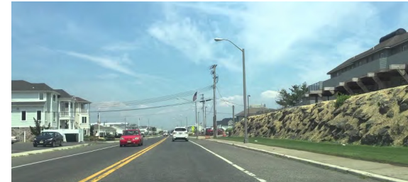
Seawall, Ocean Ave
