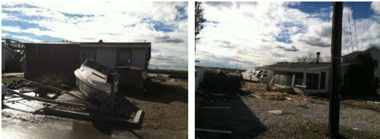
Figure 1: Aftermath of Superstorm Sandy Photo Credit: Stafford Township, Hurricane Sandy 2012 Photo Gallery
