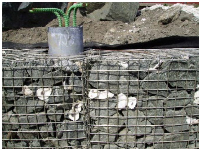
Figure 9: Gabion baskets used at Harlem River. Source: https://harlemriverpark.weebly.com/gallery.html Photo by: Thomas Lunke
