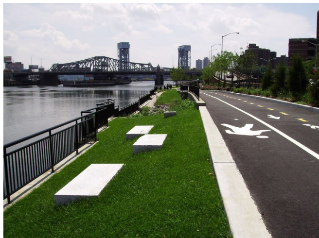
Figure 23: Terracing used to reduce slope in a space constrained environment. Figure 21: Terracing used to reduce slope in a space constrained environment. Source: https://harlemriverpark.weebly.com/gallery.html Photo by: Thomas Lunke
