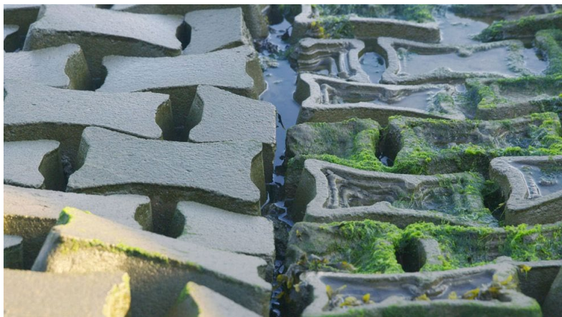
Figure 22: Effect of using enhanced concrete and surface texture to enhance habitat. Source: https://econcretetech.com/blogcat/ecological-concrete-block-mattresses-acbm-scientific-study/
