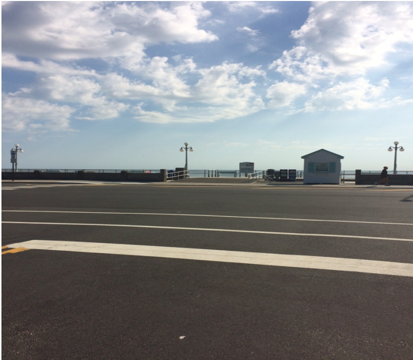
Figure 1: Avon-by-the-Sea Boardwalk, located on Ocean Avenue.
