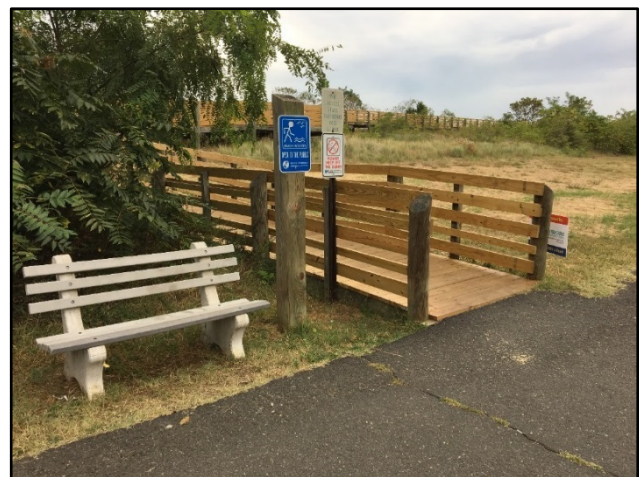
Figure 20. ADA Ramp to the Baywalk East (Site 29)
