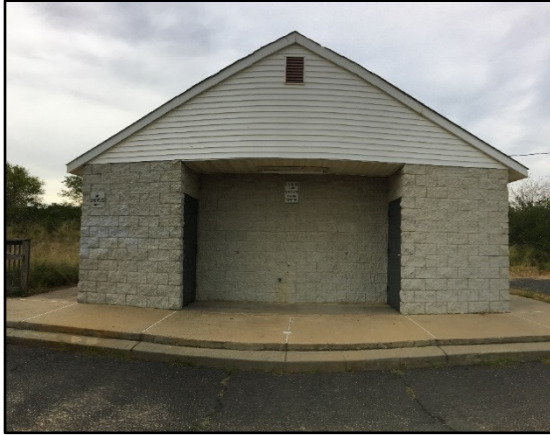
Figure 16. Public Bathroom Building
