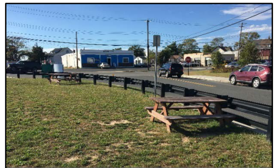
Figure 4. Picnic Area at Waackaack Creek Bulkhead
