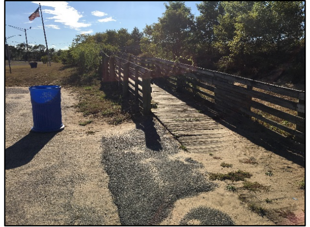
Figure 10. Ramp to the Baywalk West Boardwalk (Site 8)
