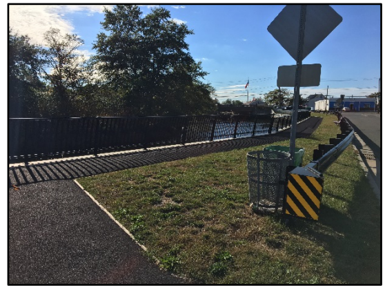
Figure 2. Waackaack Creek Bulkhead
