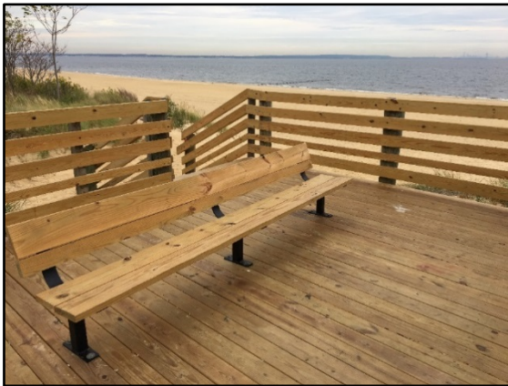
Figure 22. Beach Access Point 30
