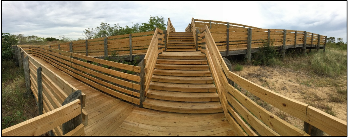
Figure 21. ADA Ramps and Stairs at the Baywalk East (Site 29)
