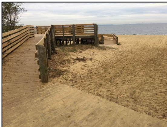
Figure 24. Beach Access Point 32
