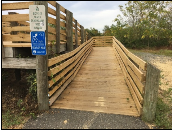
Figure 26. ADA Ramp at Baywalk East (Site 34)
