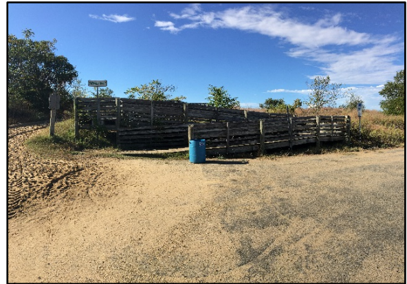
Figure 6. Western Terminus of the Baywalk West Boardwalk (Site 4)
