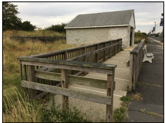
Figure 15. ADA Ramp at the Public Bathroom Building
