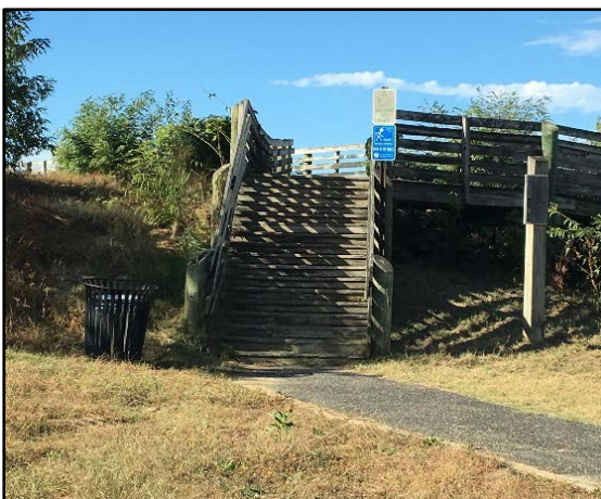
Figure 7. Stairs to the Baywalk West Boardwalk (Site 7)
