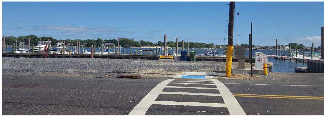
Figure 2: Marina facilities at the Shark River Municipal Marina.
