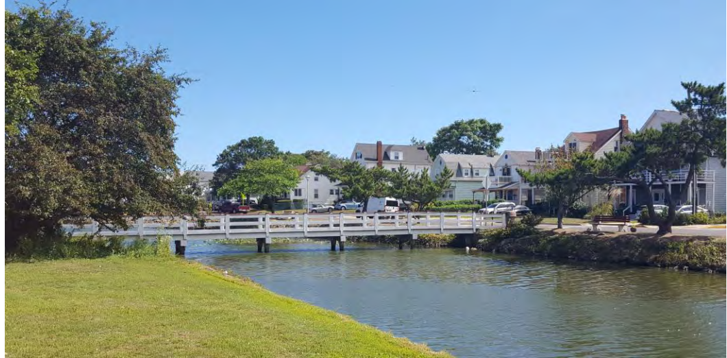
Figure 3: Bridge at Fletcher Lake
