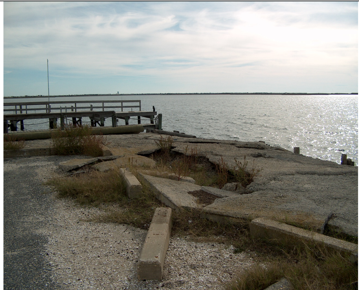
Severe Superstorm Sandy Damage at Benny's Landing
