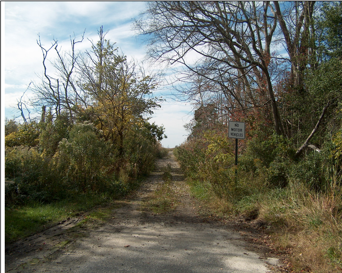
End of Improved Section of Goshen Landing Road
