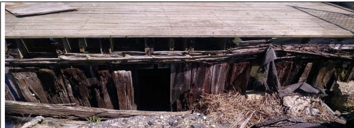
View of Collapsed Bulkhead Looking onto Pier
