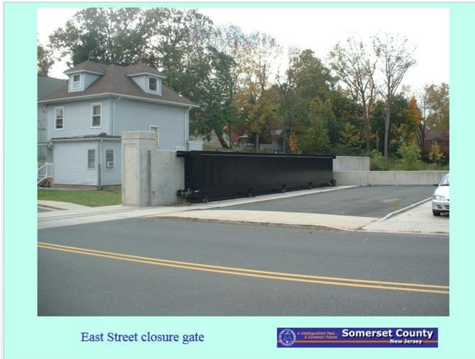
Fig.B7 Flood Gate Closure Gate (Closed Prior to a Storm Event)
