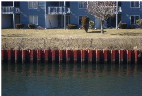
(a) Steel Bulkhead along the Pt. Pleasant Canal
