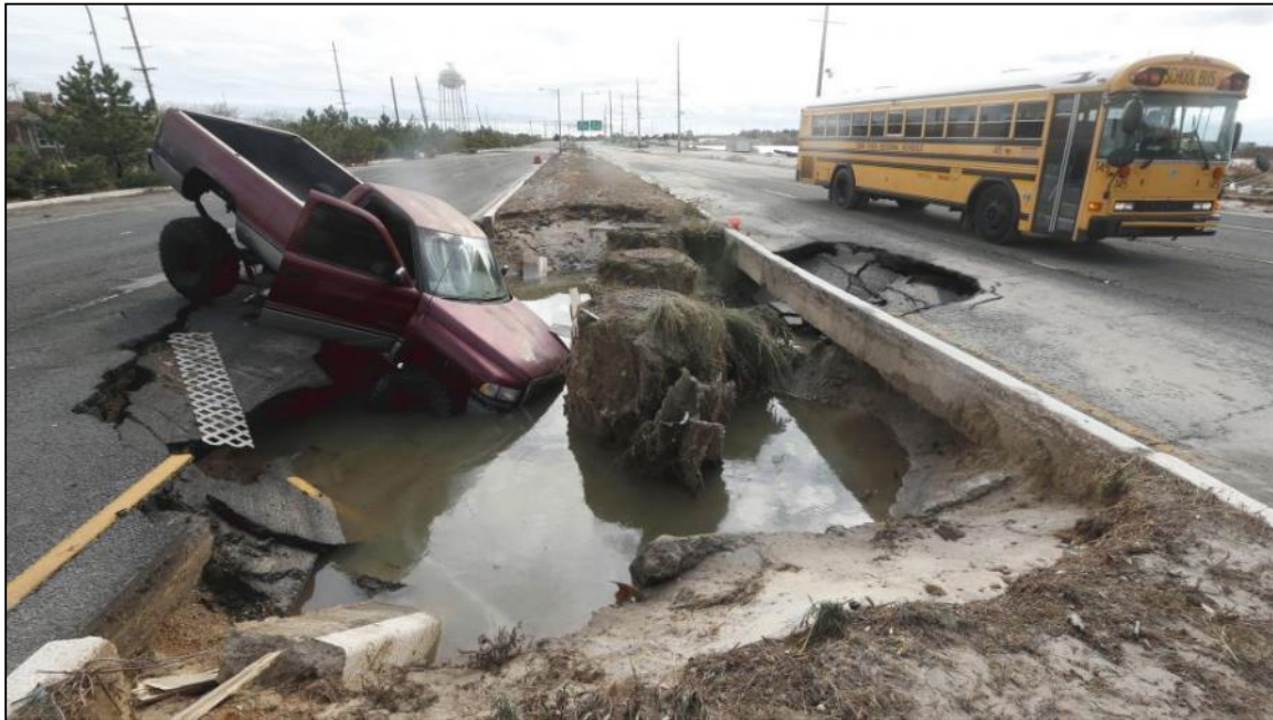
Fig. 1.3 Superstorm Sandy Damage to the Infrastructure, Seaside Heights, New Jersey (AP Photo/Julio Cortez)
