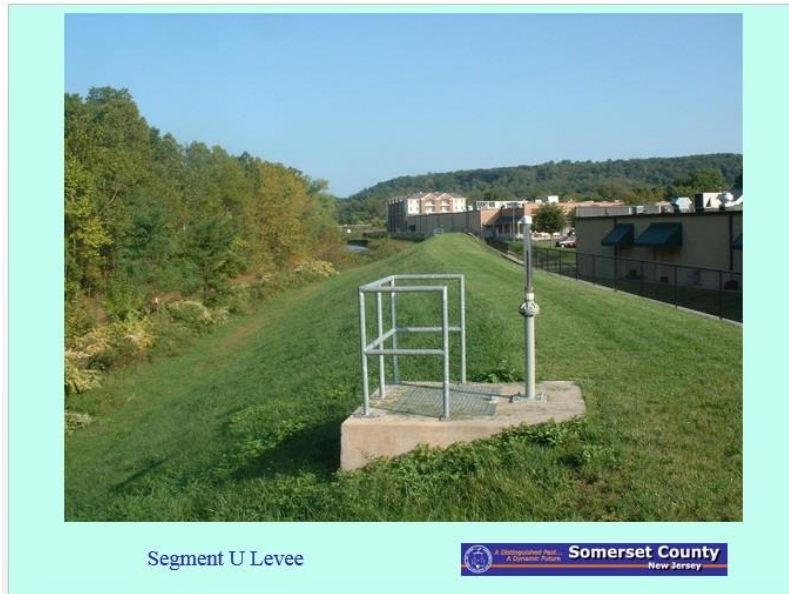
Fig. B8 Vegetated Earthen Levee
