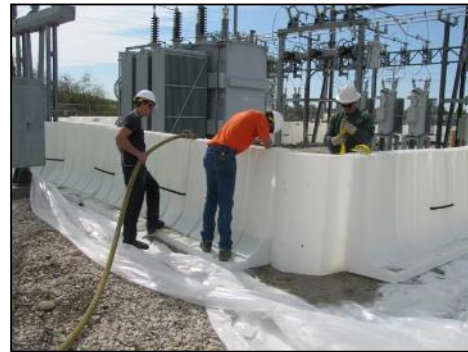
(b) Protecting Infrastructures/Utilities
