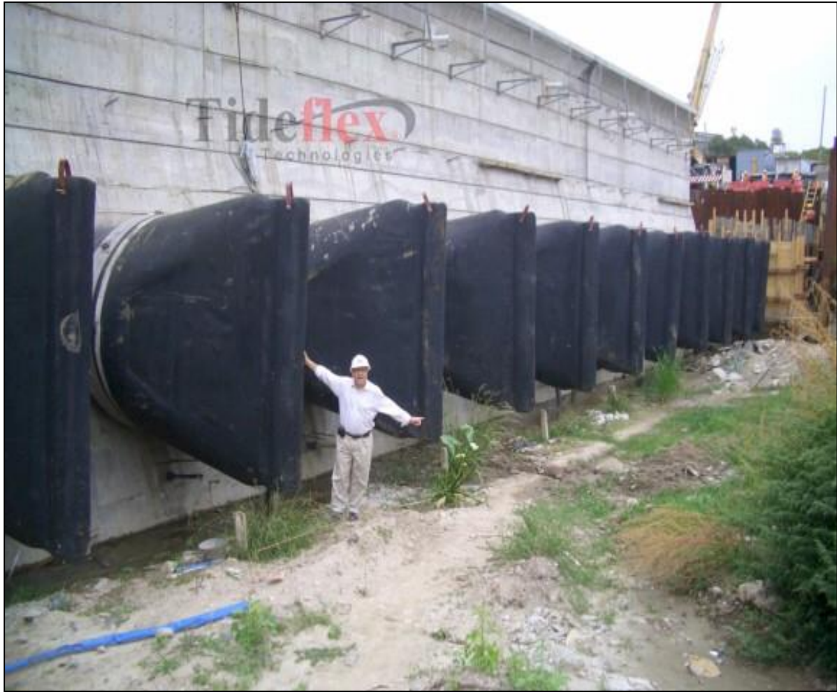
B12.2 Check Valve Used for Backflow Prevention (Source: http://www.tideflex.com/tf/index.php/content/view/228/368/ )
