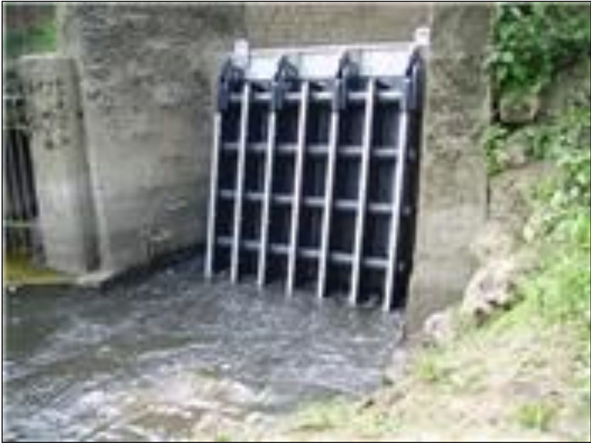
Fig. B12.1 Flap Valve Used to Prevent Backflow (Sources: http://www.hcwatercontrol.com/Flap-Valves )
