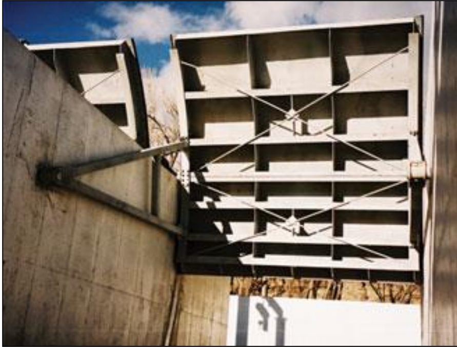
Fig. 4.10.2 Radial Gate (Source: Golden Harvest, Inc.) ( http://www.goldenharvestinc.com/products/ )
