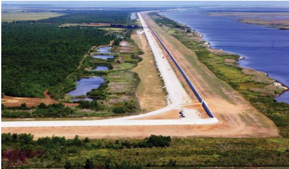
Fig. B11.3 Concrete Floodwalls on Earth Levees
