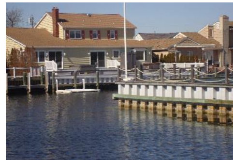
(a) Steel Bulkhead along a Dredged Lagoon
