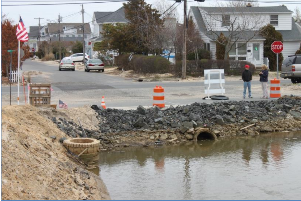
Fig. 2.2 An Outfall of a Storm Sewer at a Normal Tide Elevation in Seaside Heights, New Jersey Showing the Storm Sewer is about Half Full of Water (photo taken in April 2013).
