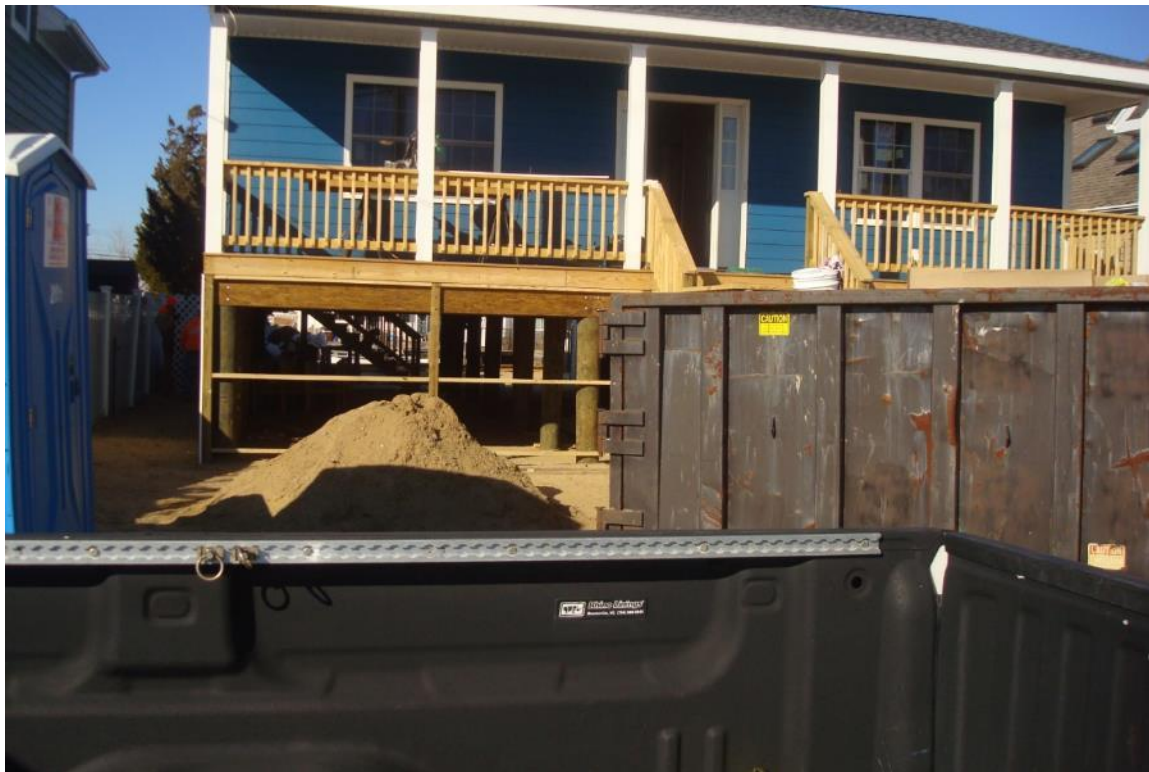
Fig.4.8.3 Elevating a Residence in Progress at Seaside Heights Borough, NJ
