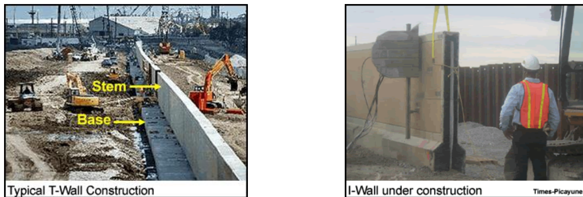
Fig. B11.2 Flood Wall Under Construction ( http://library.water-resources.us/docs/MMDL/FLD/Feature.cfm?ID=2 )
