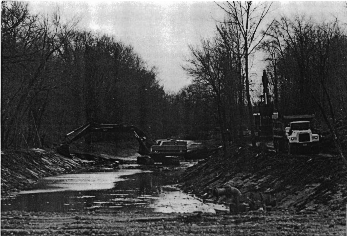
Alexander Road, Princeton. In 1984-85 the Water Supply Authority removed 650,000 cubic yards of silt from the canal. It was the most comprehensive dredging project of the century for the D & R. As a result the canal flows more freely, making it a far better water supply system, recreation site, and fish habitat.
