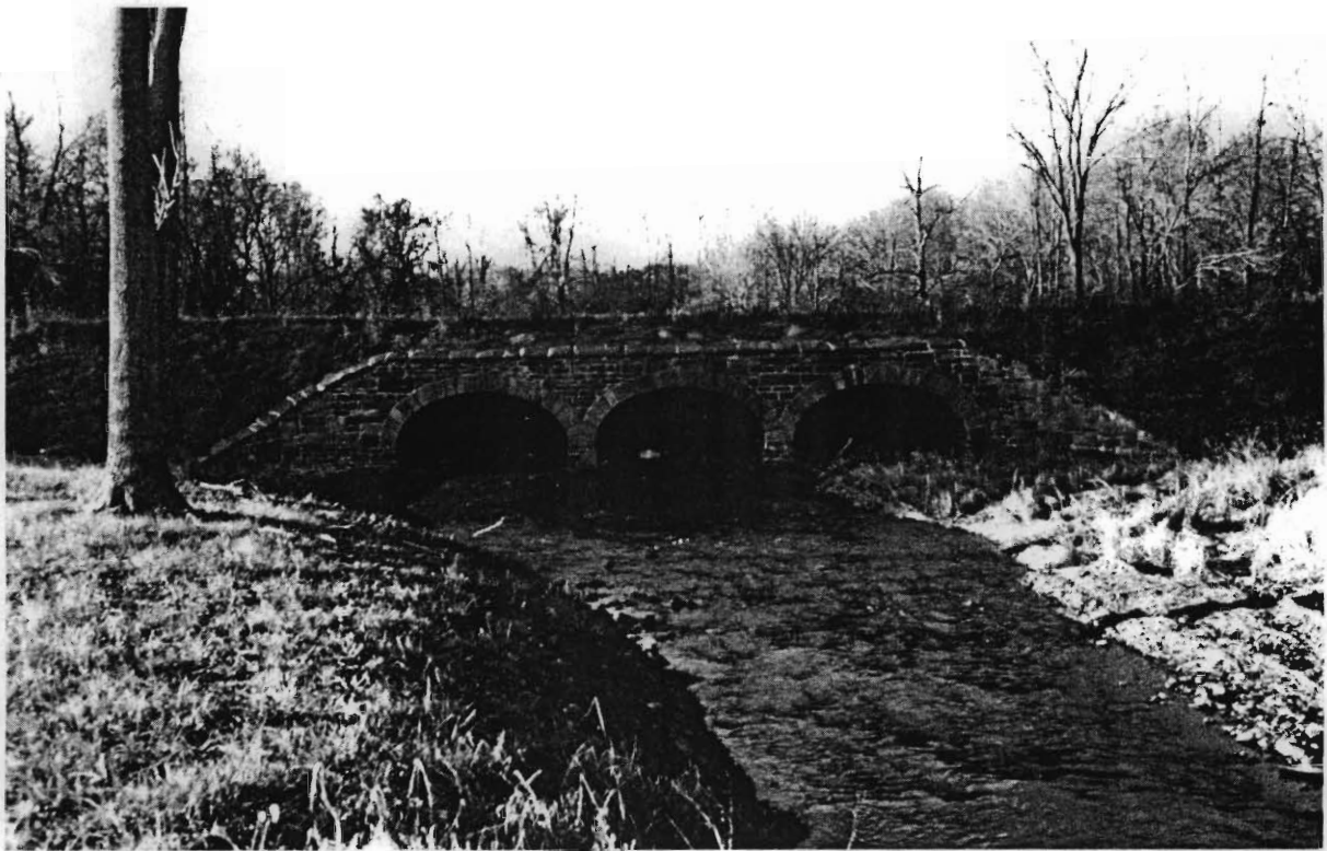
Ten Mile Run Culvert, Franklin Township. Many streams are directed under the canal in culverts that were built in 1831-34 when the canal was constructed. The Ten Mile Run Culvert was recently rehabilitated.
