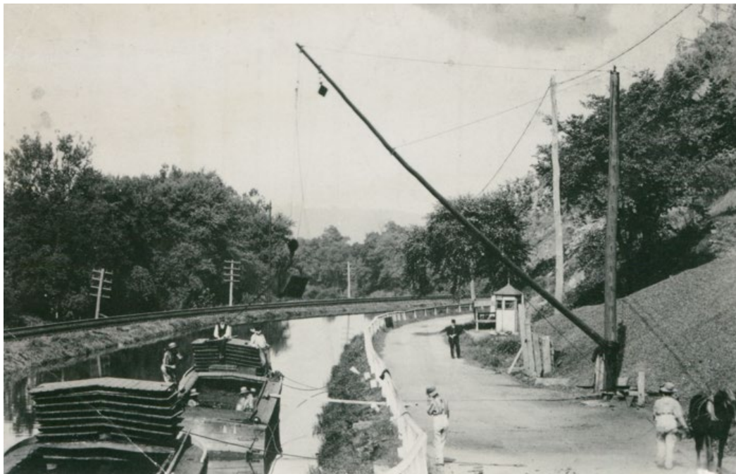
(Coal is unloaded using a pole boom from canal hinge boats at the Mercer County Workhouse, circa 1900. Note the armed guard sitting on hatch supervising the work.)
