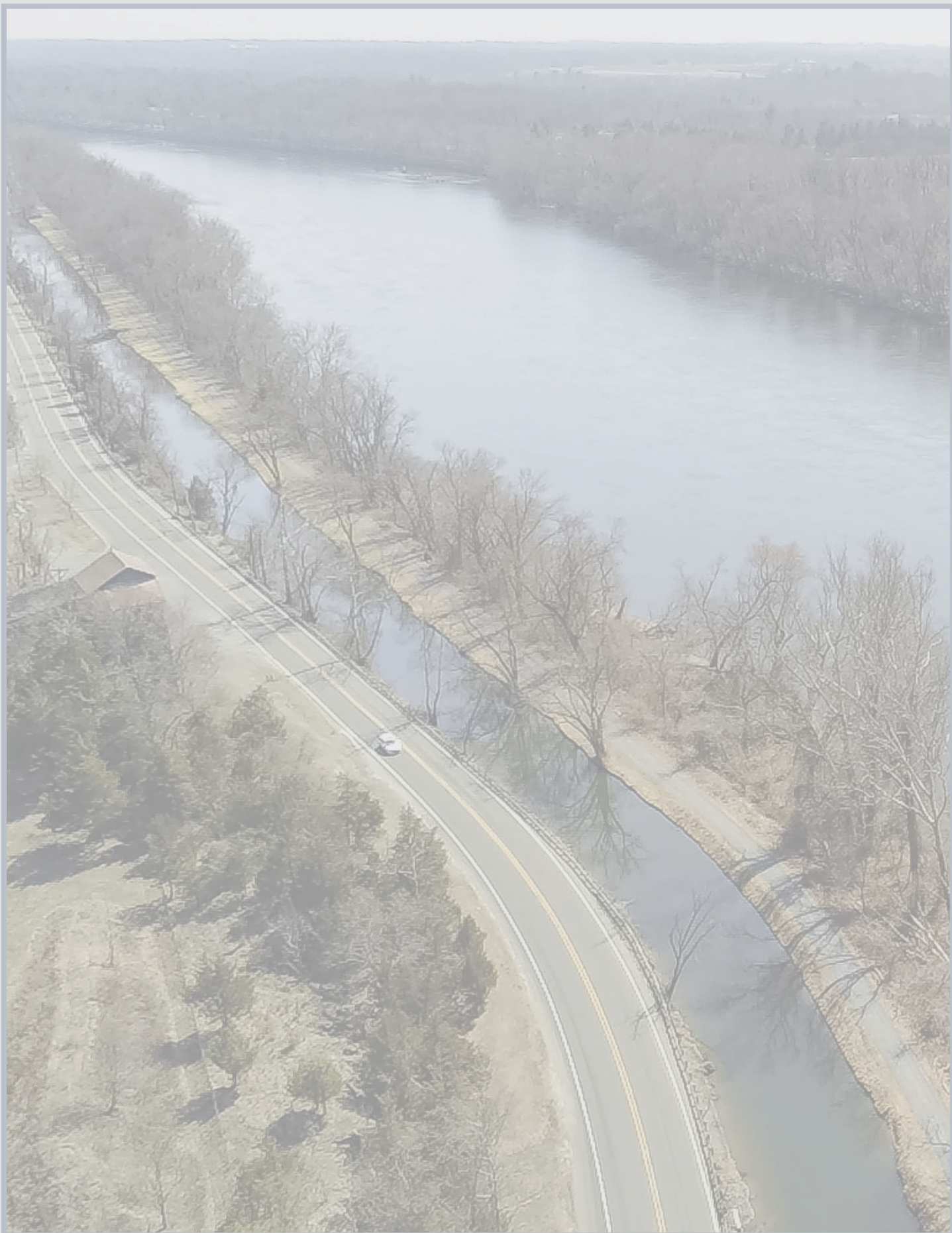
On the cover: Southern view of the D&R Canal, alongside Route 29, in Hopewell Township, Mercer County. Drone Photo: Steven Jacobus
