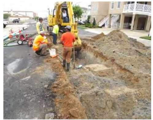
North Wildwood Sewer, Storm and Street Restoration
