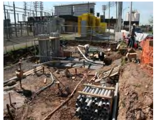
Passaic Valley Sewerage Commission Electrical Substation
