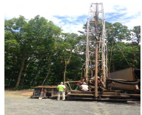
Drilling of a Drinking Water Well at the Berkeley Twp. MUA
