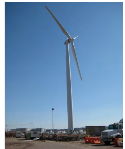
Bayonne MUA Wind Turbine for a Pump Station
