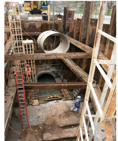
Passaic Valley Sewerage Commission Interceptor Slip Lining
