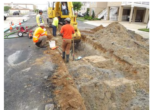
North Wildwood Sewer, Storm and Street Restoration
