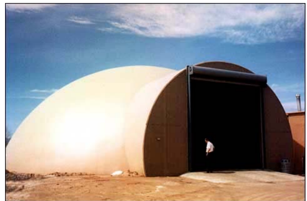
Monolithic, or shotcrete dome.
