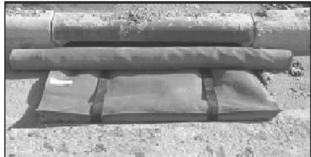
Storm drain inlets blocked during bulk fuel transfer.
