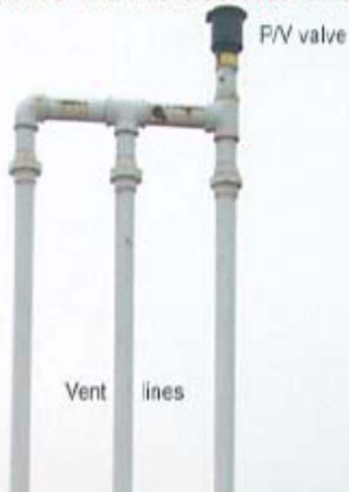
Three vent lines manifolded into one.
