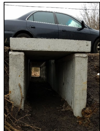
An under-road tunnel on the Assunpink WMA.
