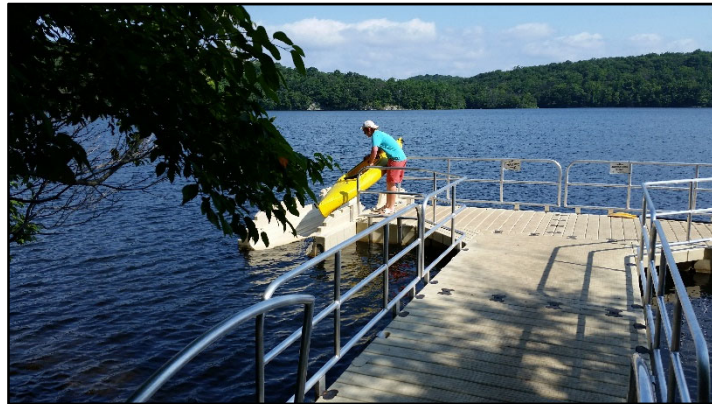
One of the newly installed docks at the Split Rock Reservoir.
